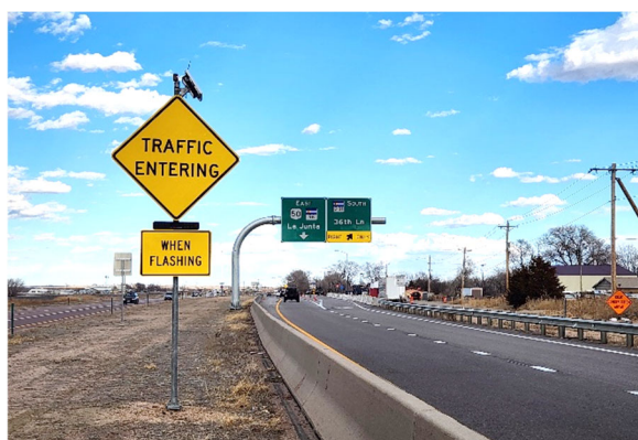
Warning on Eastbound US 50 Approach
