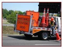
Work Zone Removal – Ideally, the work zone is removed in the opposite direction of set-up; downstream to upstream leaving the first warning sign the motorist sees as the last item of protection picked up by workers.
