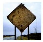
When signs are not in use, it is required that they be taken down or fully covered. Sign covers are detailed in the CDOT Specifications manual. Sign covers may be made of durable plastic, wood, metal, or polypropylene. Signs which are taken down or faced away from traffic, must be stored outside of the clear zone.
