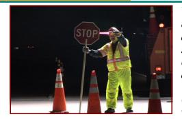
Work Zone Nighttime Operations – Nighttime operations are considered to be operations conducted between sunset and sunrise. Consideration should be given to having night work illumination equipment in place one half hour prior to sunset and left in place until one half hour after sunrise. More and more projects are required to be completed at night for traffic volume considerations. Several issues arise in set-up of TCP's
