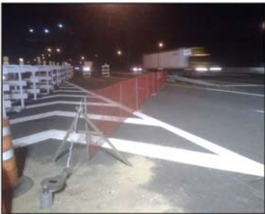
Figure 5. Vehicle Arresting System Protecting Closed Highway Section
