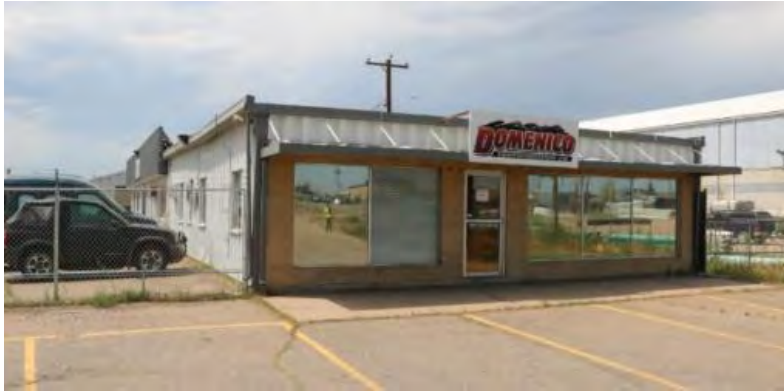
Figure 1. Photo of 5AM.4046 main building view northwest, courtesy Mead & Hunt 2019.
