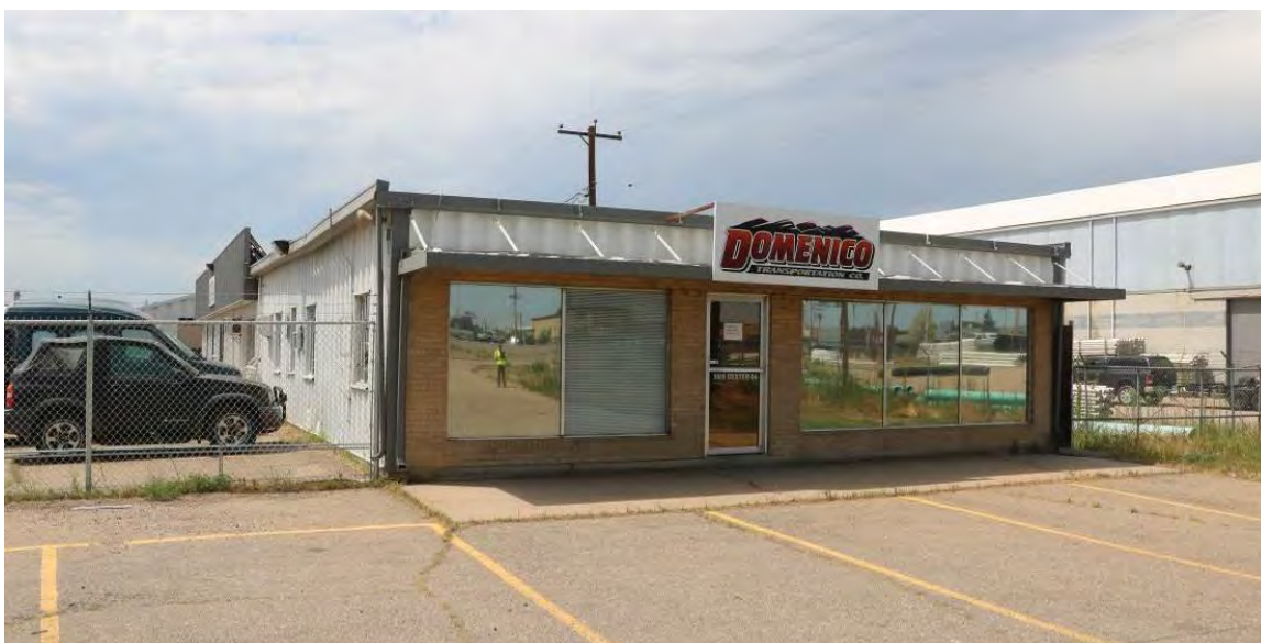
Figure 2. Building A, front (east) facade and side (south) elevation. View facing northwest.
