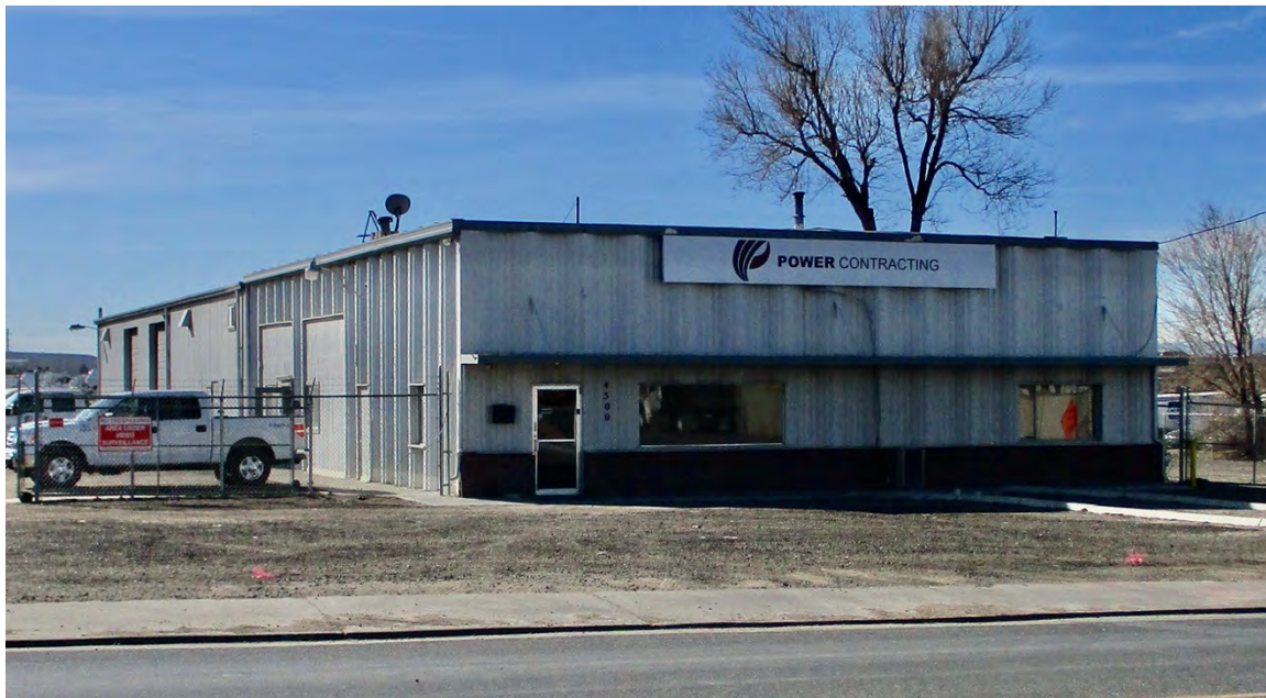
5AM4073_1.jpg: Looking south at 5AM.4073 from E. 60 th Ave. (January 24, 2020)
