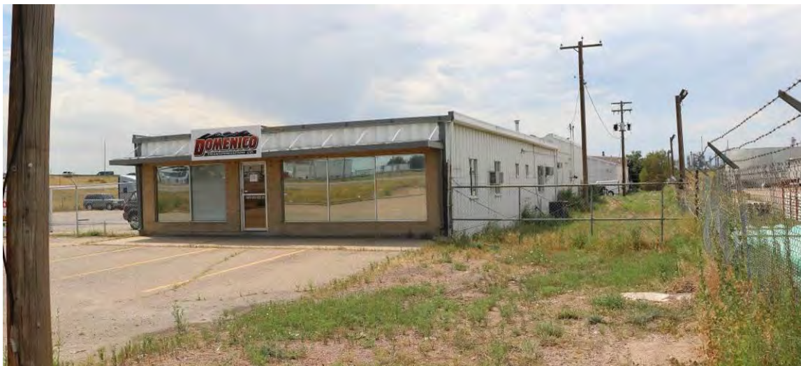
Figure 1. Building A, front (east) facade and side (north) elevation. View facing southwest.
