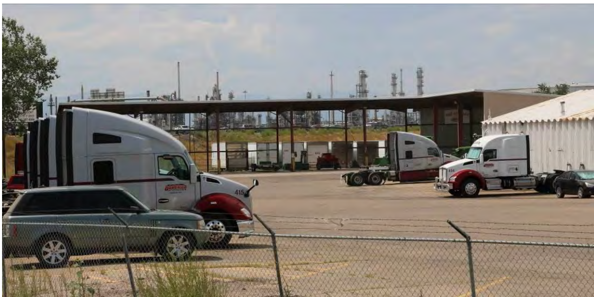
Figure 4. Building C, at left of image in relation to Building B at right. View facing northwest.
