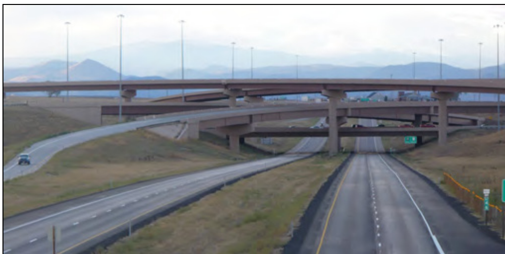
Figure 2-18. Profile View of the Four-Level Stack Interchange at I-25, E-470, and the Northwest Parkway
