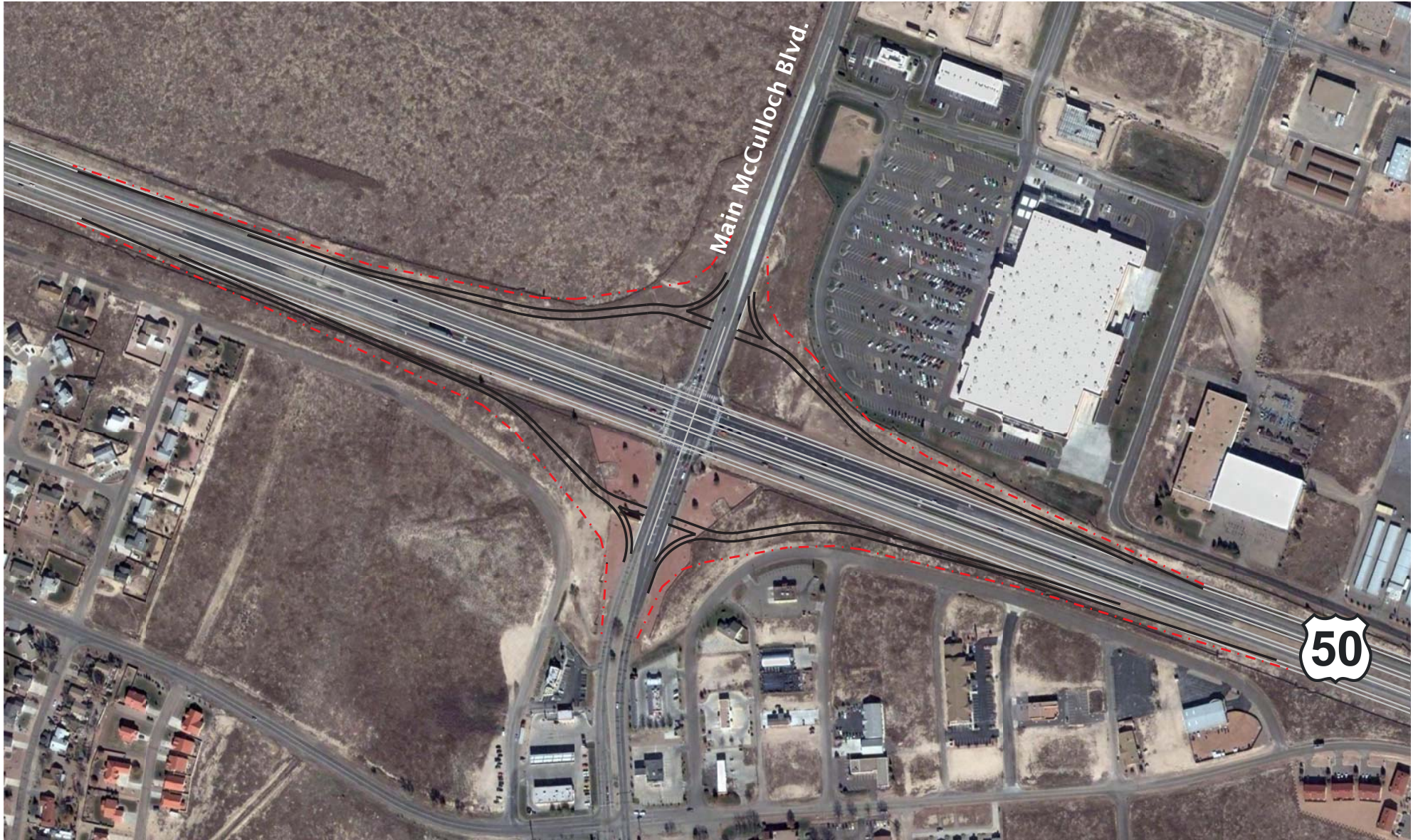
Figure 2-28. Aerial View of Diamond Interchange at Main McCulloch Blvd.
