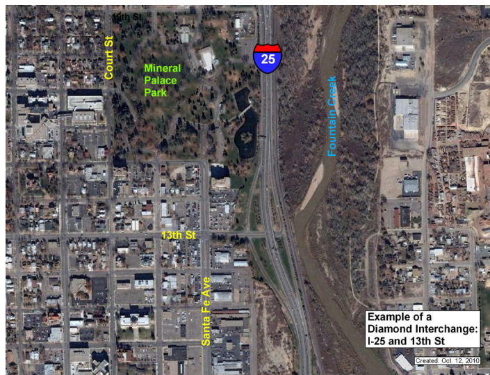
Figure 2-12. Aerial Photo of the Diamond Interchange at I-25 and 13th St. in Pueblo
