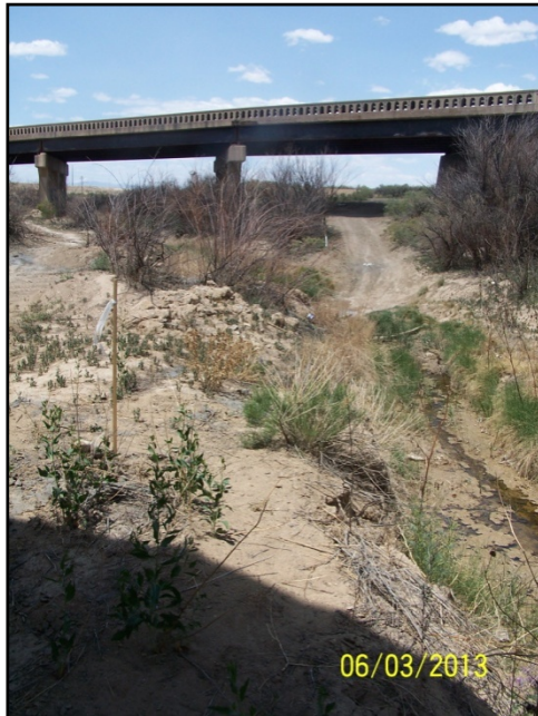
Photo 10 — Looking north from under the eastbound bridge.
