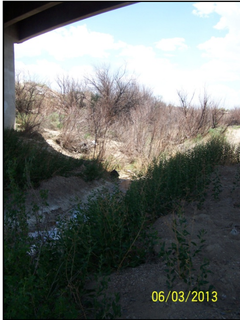
Photo 9 — Looking south from under the eastbound bridge.
