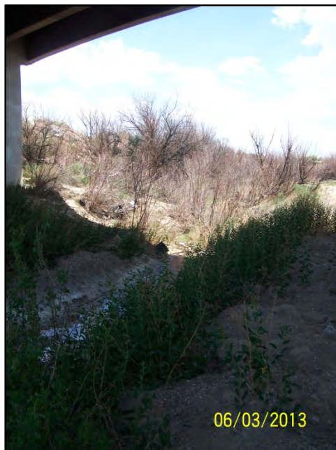
Photo 10 — Looking south from under the eastbound bridge. This channel is very narrow and filled with noxious weeds.
