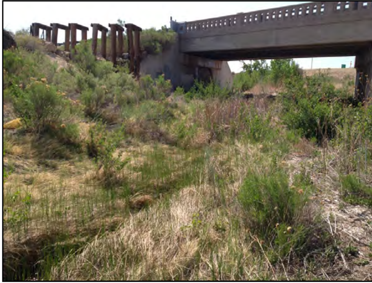
Photo 1 — Wetland WCN-1 in the background and Wetland WCS-1 in the foreground.
