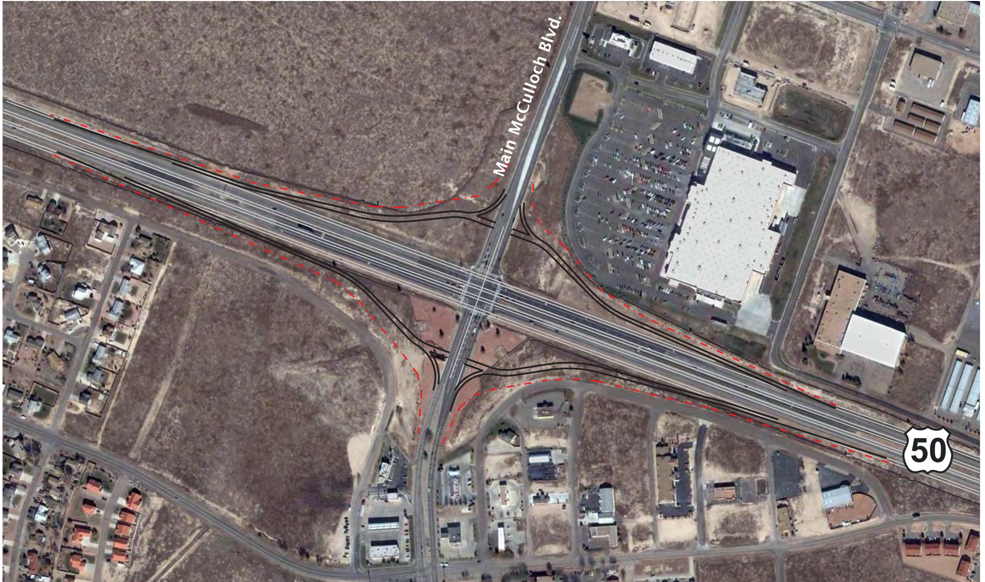
Figure 2-28. Aerial View of Diamond Interchange at Main McCulloch Blvd.
