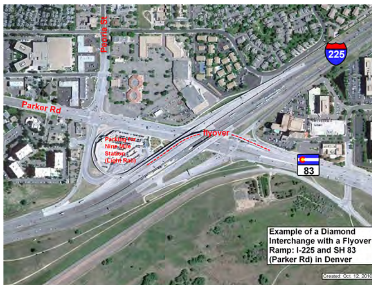
Figure 2-13. Aerial Photo of a Diamond Interchange with Flyover Ramp at I-225 and SH 83 in Denver
