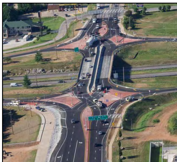
Figure 2-24. Aerial View of a Diverging Diamond Interchange in Springfield, Missouri
