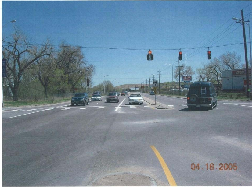
Looking east at 26th Street intersection with US 24
