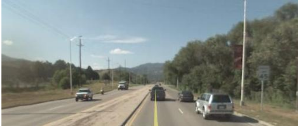
Looking west on US 24
