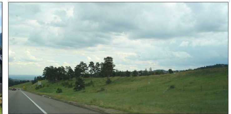
C | Where possible, earthwork and landscaping should be utilized to buffer community-based land uses from the corridor rather than stand-alone soundwalls.
