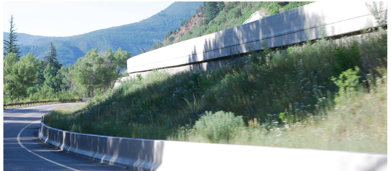
C | Continuous concrete barriers with a consistent color application should be utilized rather than segmented barriers.
