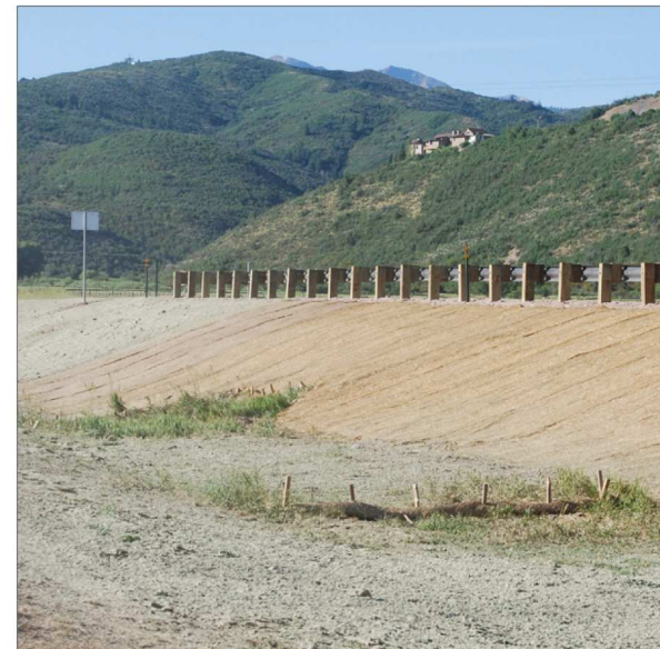
B | Utilize soil retention blankets, mulches, and other revegetation techniques that improve the chances of successful re-establishment.
