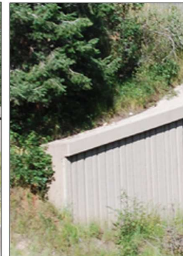
D | Turning the ends of walls helps integrate them into the adjoining slope.
