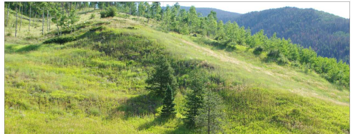
D | Utilizing variable slopes through the length of an embankment mimics the natural patterns.
