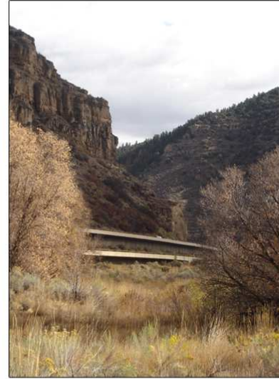
A | Using a split elevation for the travel lanes will adapt the corridor to the steep slopes found in this segment.
