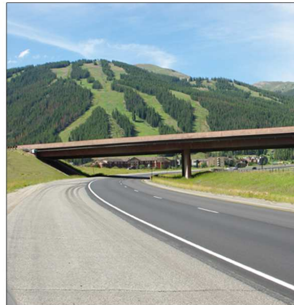
B | The bridge at Copper Mountain presents an aesthetic character with color, shadow, and box girder construction.
