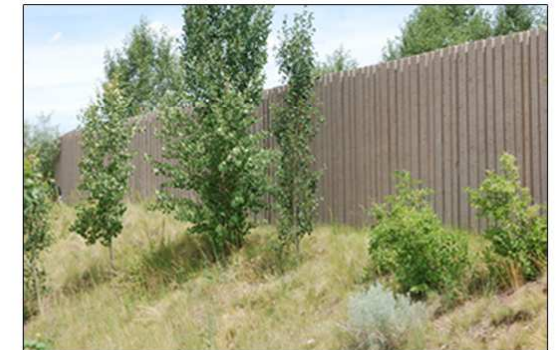
E | When sound walls are required, utilize berming, landscape, texture, and limited wall height.
