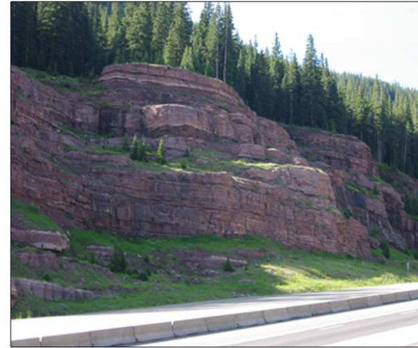
A | Rock cuts should include naturalized benches with planting pockets to mimic the surrounding landscape.
