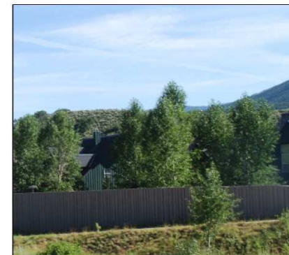
B | This community interface successfully uses a combination of landforms, walls, and planting solutions for noise reduction.
