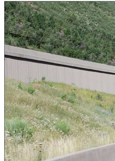
C | Incorporate earthwork solutions in conjunction with retaining walls in order to limit retaining wall height.
