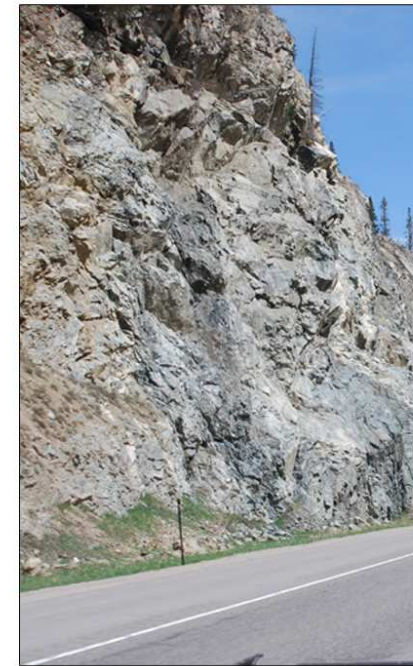
D | Color staining techniques will blend new rock cut with existing rock features.
