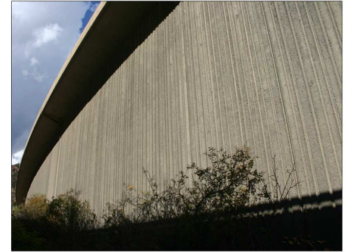
B | Simple vertical textures provide depth and shadow to large wall faces.
