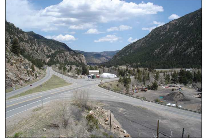
B | The interchange at Empire Junction houses a maintenance yard.
