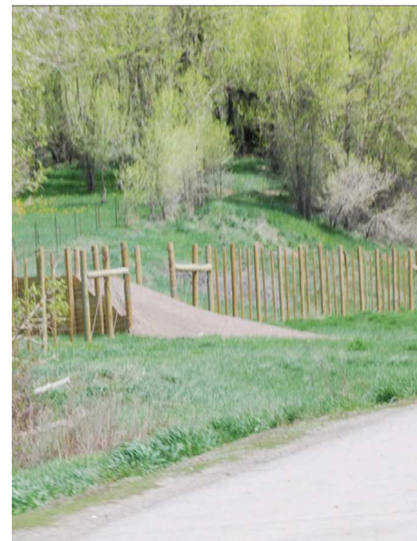
C | Fencing constructed with pressure treated posts will weather and blend into the landscape.
