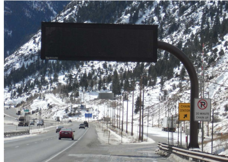
A | Single arm-monotube systems should be used.
