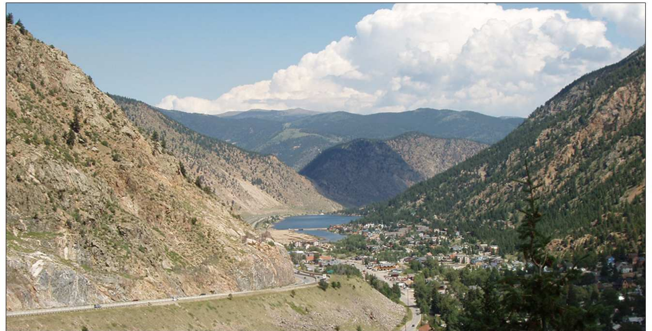
C | Road service areas should be designed to highlight and preserve site resources and scenic views.
