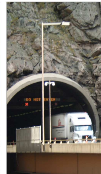
B | Light poles should be of an elegant and simple design with full-cutoff luminaire fixtures. The image on the left is an ideal example.
