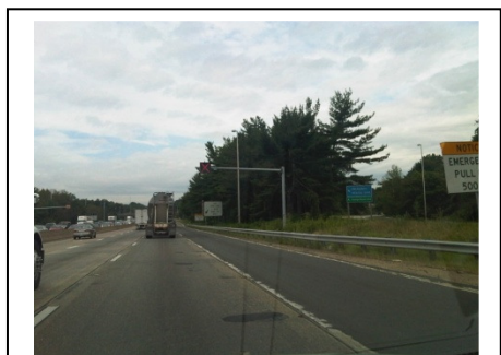
The hard shoulder concept allows vehicles to travel on existing shoulders during limited time periods, resulting in additional roadway capacity to manage congestion.
