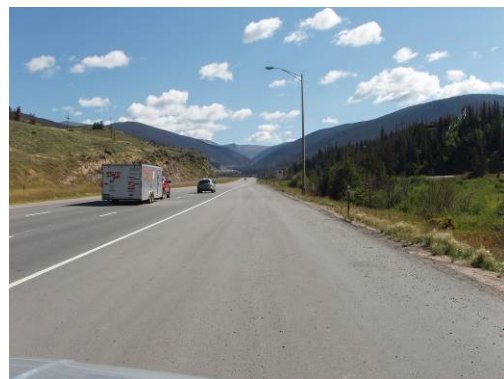
EB MP 205 Chain Station
