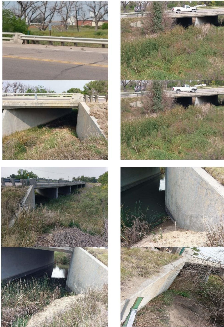
Figure 8. Bridge C 22 BS Pictures
