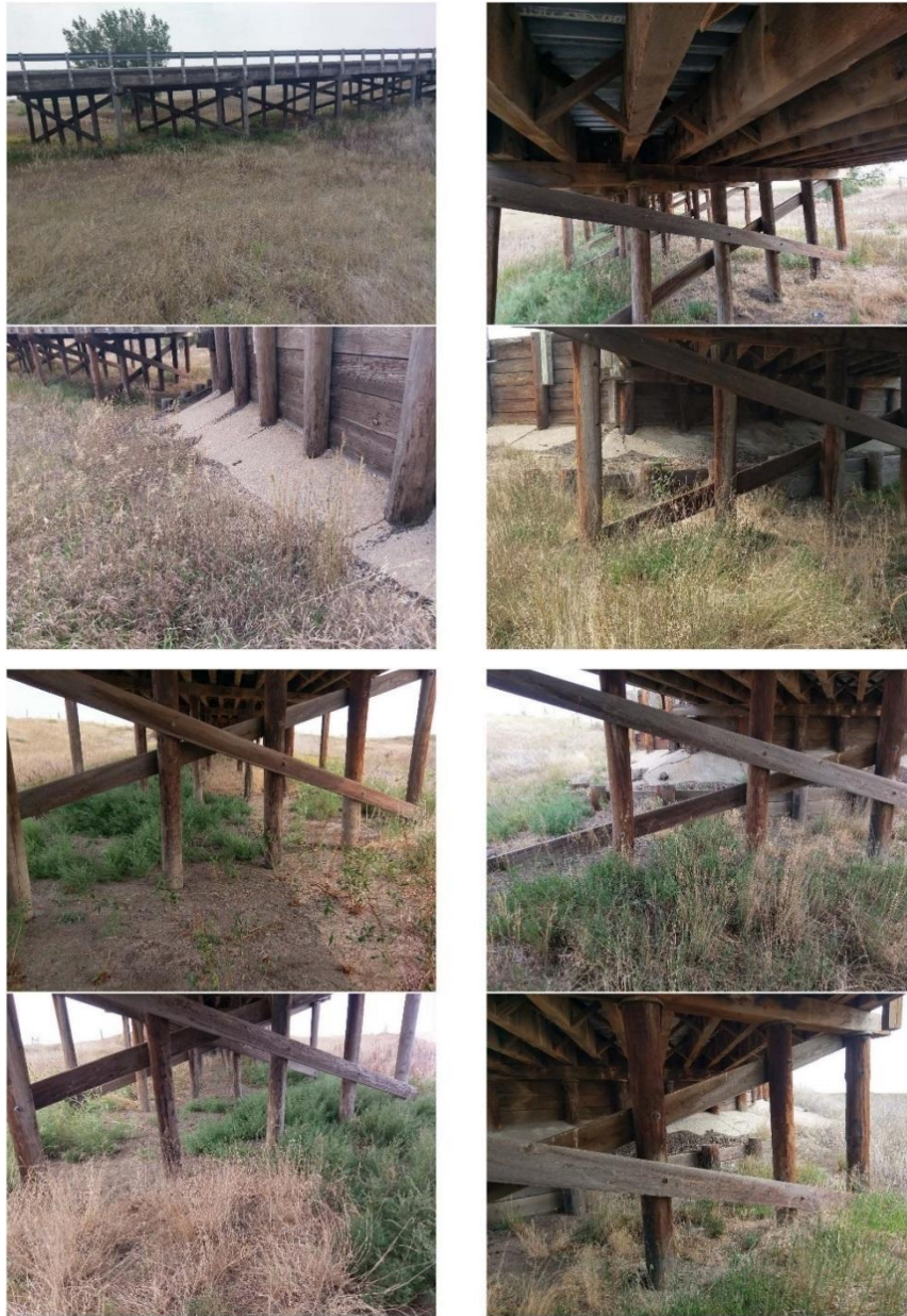
Figure 6. Bridge D 22 C Pictures
