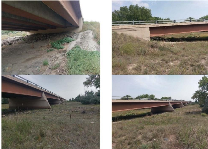
Figure 10. Bridge C 22 BT Pictures
