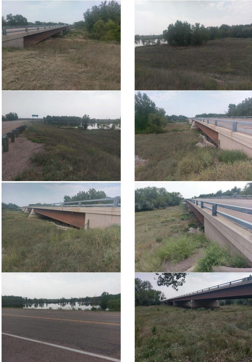
Figure 9. Bridge C 22 BT Pictures
