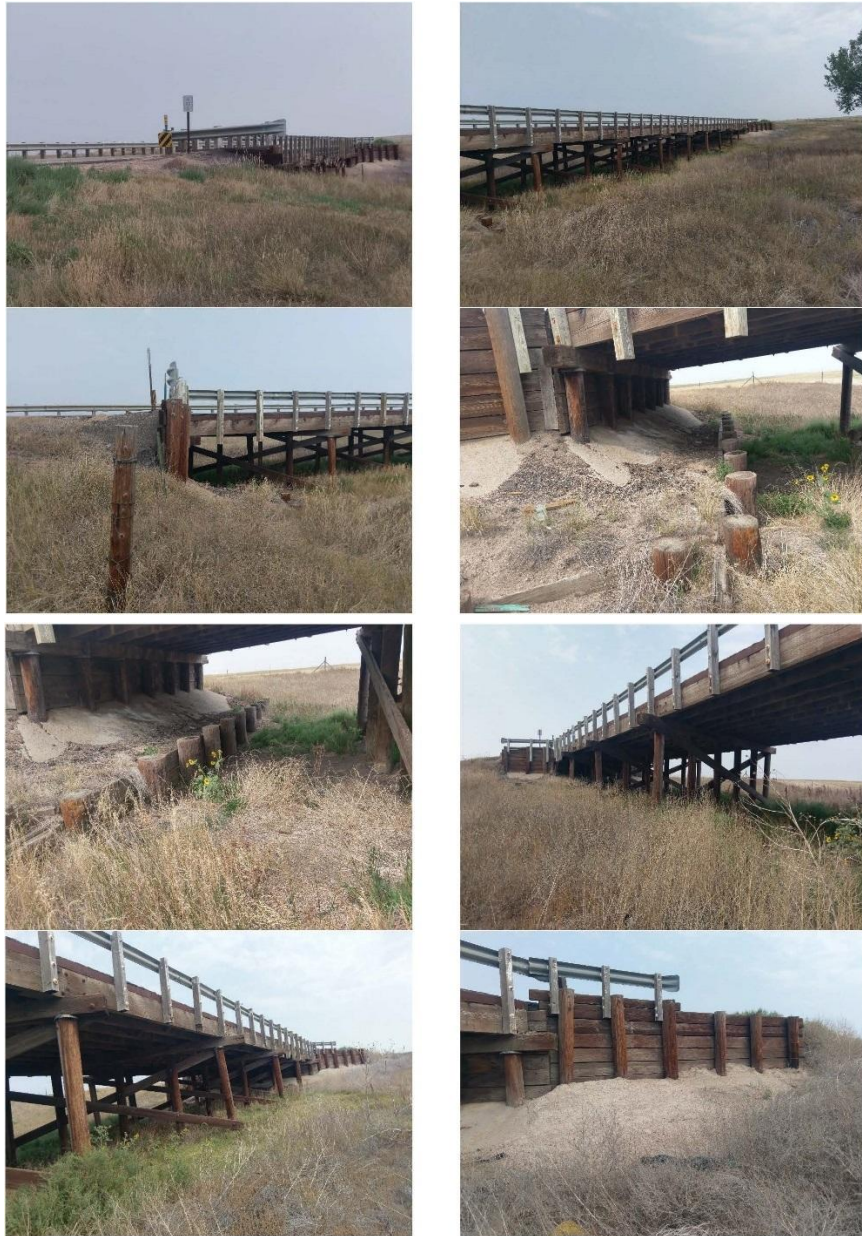
Figure 4. Bridge D 22 C Pictures
