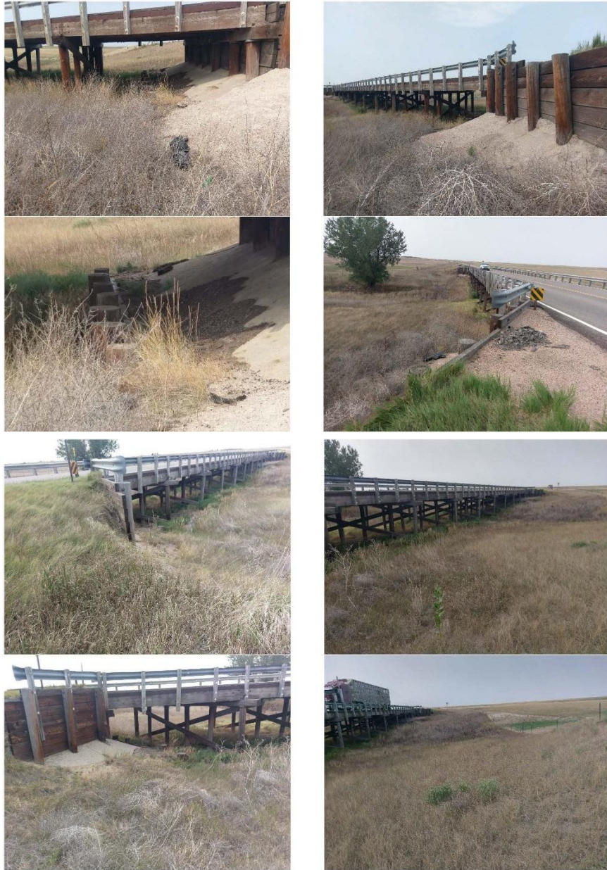
Figure 5. Bridge D 22 C Pictures
