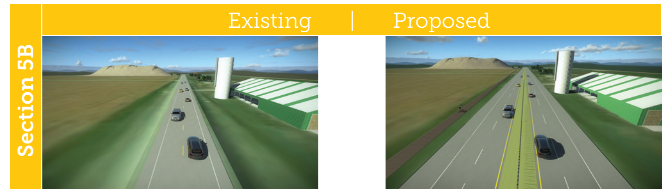
No median separation or left turn lanes
