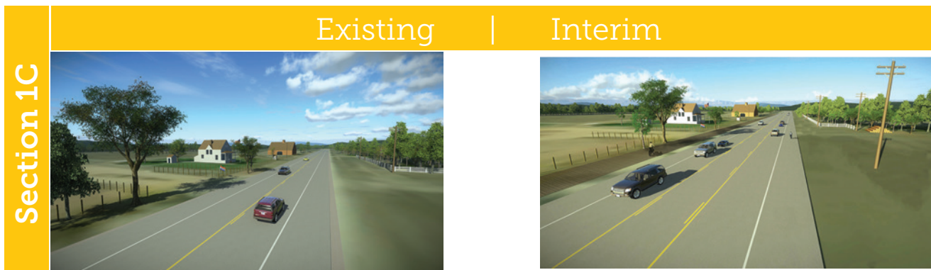
No median separation or left turn lanes
