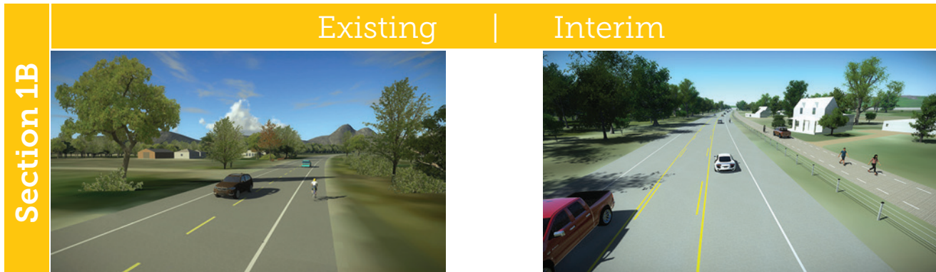
No median separation or left turn lanes
