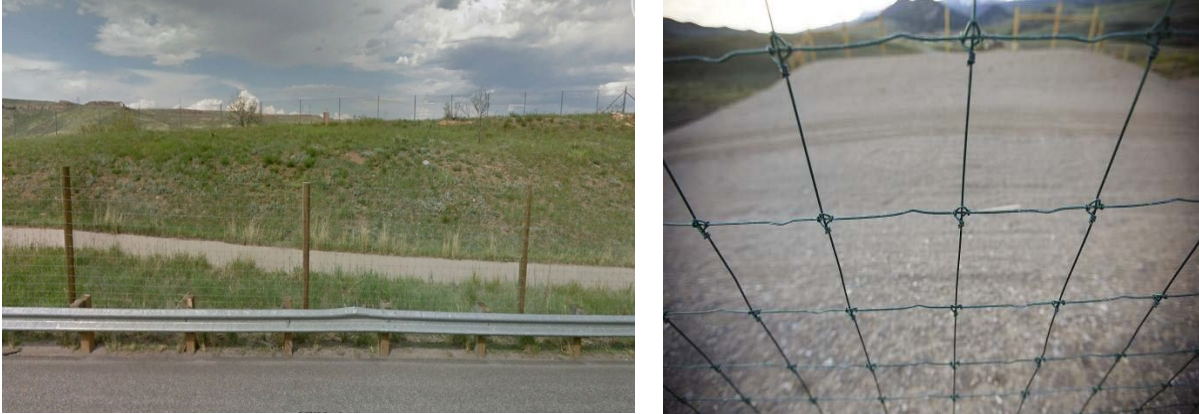
Figure 4-12. Photos of CDOT Standard Right-of-Way Fencing
