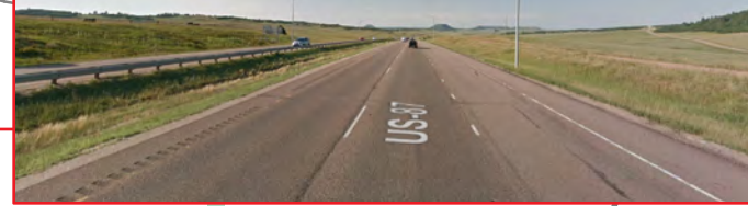
MP 163.6 NB: Galvanized pole cobra-headed lamps, Type-3 guard rails in median, and no guard rails along roadway edge.
