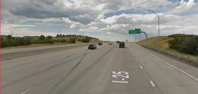
MP 188.2 NB: Monotube cantilever sign and scissor design light pole.
