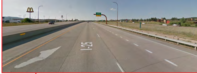
MP 161.0 NB: Start of segment. Median barrier, cobra-headed light pole and brown monotube cantilever sign.
