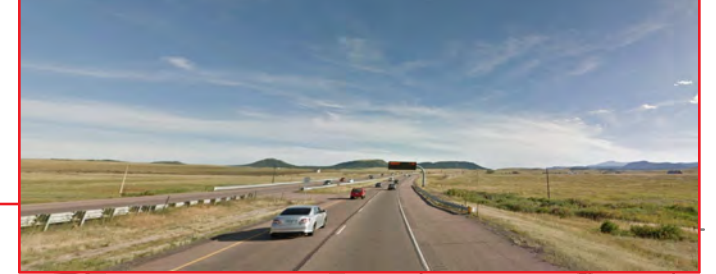
MP 167.7 SB: Galvanized monotube cantilever VMS sign and Type-3 guard rails in median and along roadway edge
