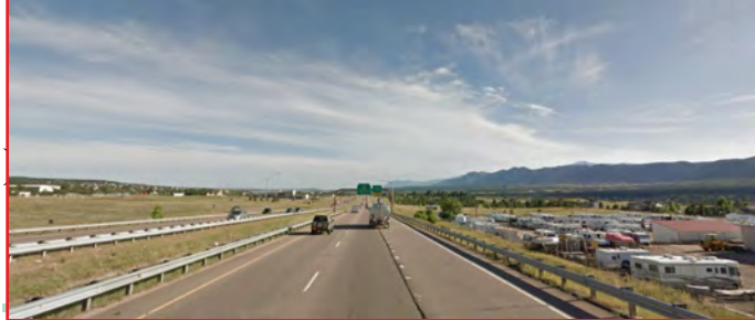
MP 162.2 SB: Brown monotube sign bridge sign and Type-3 guard rails in median and along roadway edge.
