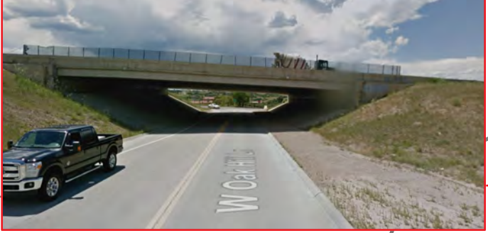
MP 189.8: View west from Oak Hill Lane toward overcrossing by I-25.
