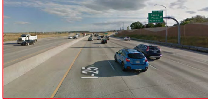
MP 188.7 SB: Concrete sound wall, cobra-headed light pole, and cantilever sign.
