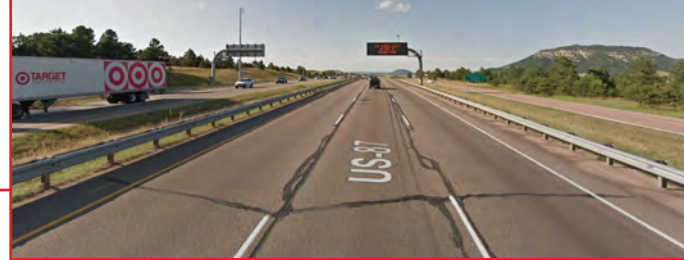
MP 162.9 NB Galvanized monotube cantilever signs and Type-3 guard rails in median and along roadway edge.
