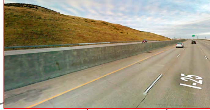
MP 191.8 NB: Smooth-surface retaining wall in median.
