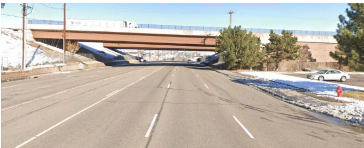
Picture: Washington Street at I-270 Looking Northbound
