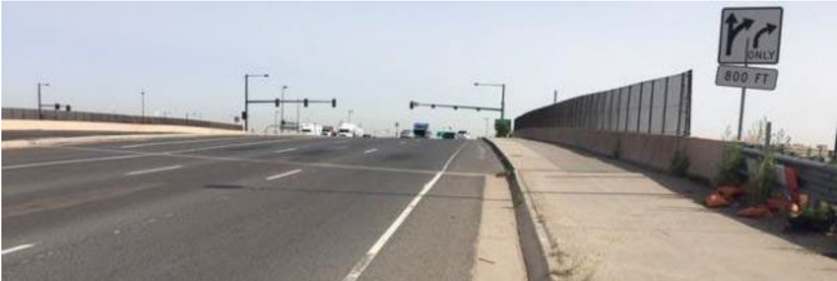
Picture: Quebec Street over I-270 Looking Northbound
