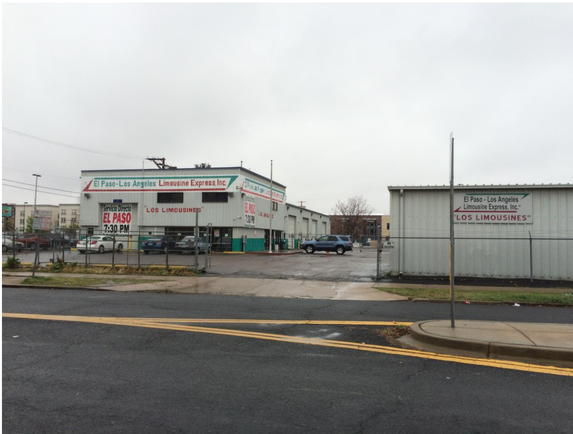
Figure 2-12: EPLA Facility as seen from 22 nd Street
