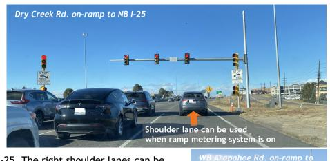
Road on-ramps to northbound I-25. The right shoulder lanes can be used when the ramp metering signals are on. The use of the part-time shoulder lanes allows more drivers to enter the interstate quicker, while preventing impacts to nearby local roads. The shoulder lanes can be used ONLY when the ramp metering system is activated.
