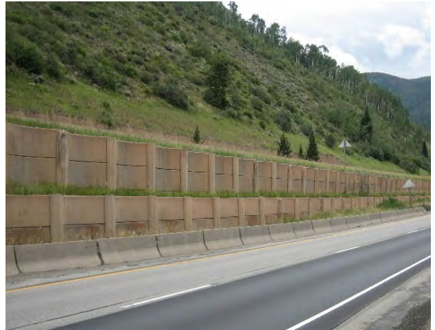
Existing Pre-cast Curved Concrete Wall
