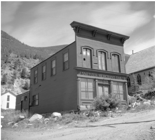
Snetzer's Tailor Shop, Georgetown. Single Storefront commercial building. Courtesy of Denver Public Library, X-1303.
