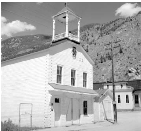
Star Hook and Ladder Firehouse, Georgetown. Courtesy of Denver Public Library, X-1299.
