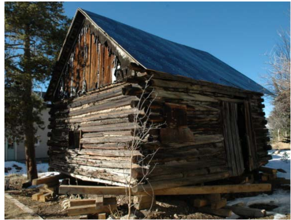
Klack Placer Cabin, Breckenridge. Source: Carl McWilliams.
