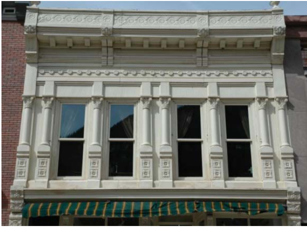
Mahr Building in Telluride, Colorado, with 1892 Mesker Bros. cast iron façade. Source: Carl McWilliams.
