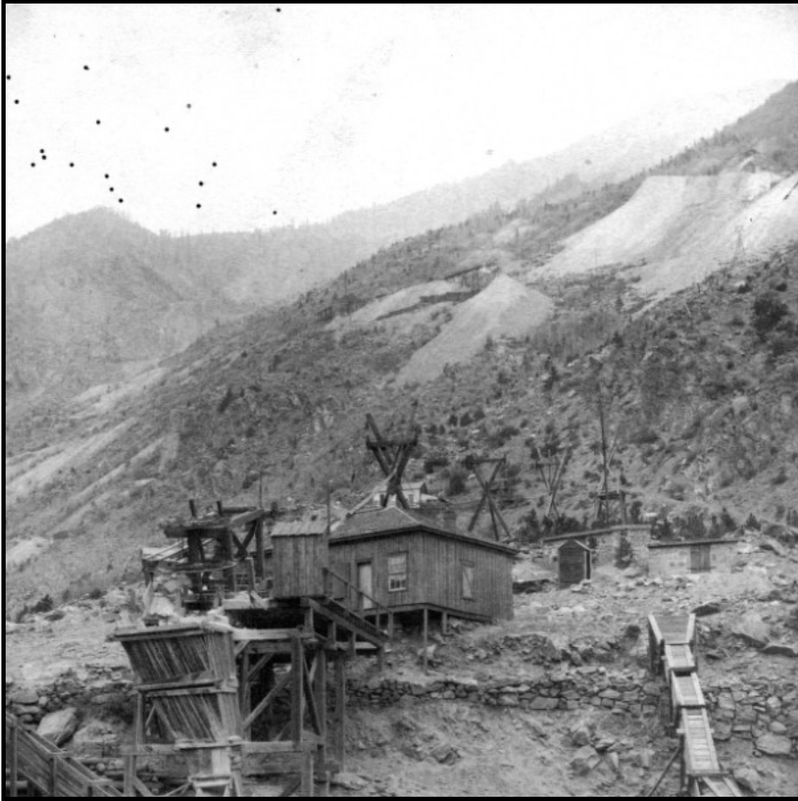
At the Pay Rock Mine near Silver Plume, a Hallidie tramway lowered ore from workings high on the mountainside down to a bottom terminal and loading station. The sheave wheel is enclosed in the slanted frame above the ore bin. The towers are unusual tripod structures. Courtesy of Denver Public Library, CHS.X4578.
