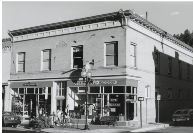
Bank Block, Idaho Springs, Double Storefront commercial building. Courtesy of Denver Public Library, AUR-981.
