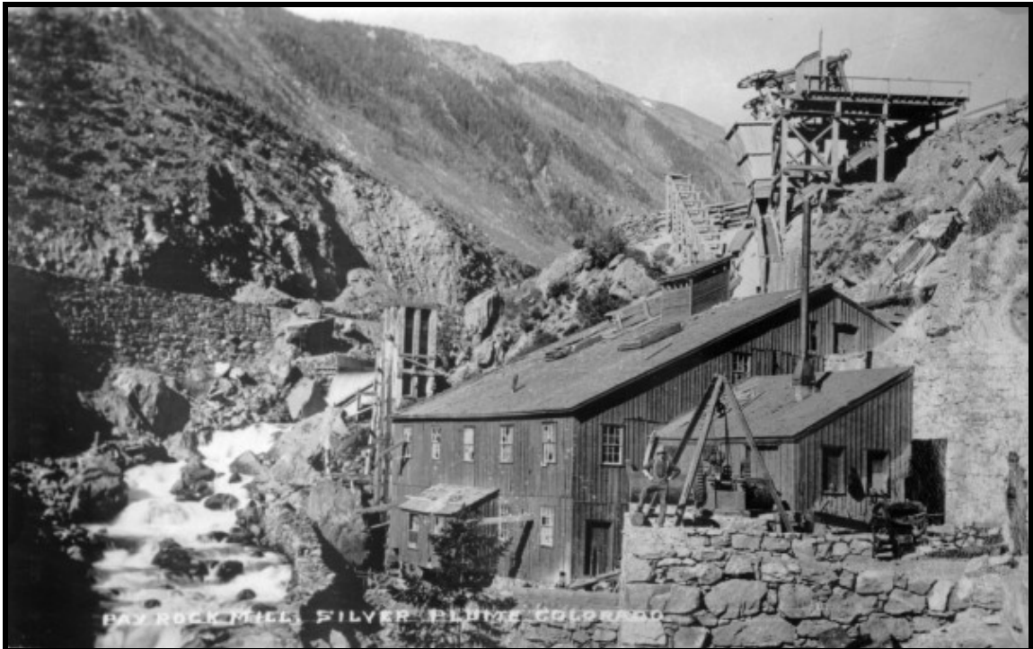
The Pay Rock Mill on the north side of Clear Creek near Silver Plume is a good example of a typical concentration facility. The building descends over a series of stairstep foundations, which are often all that remain at mill sites today. Courtesy of Denver Public Library, X-61593.
