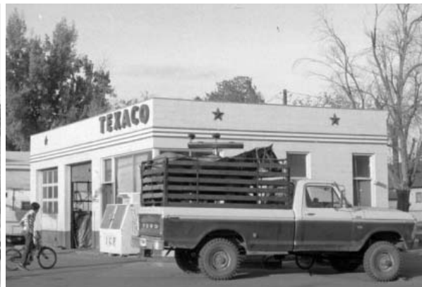
Texaco Oblong Box Gas Station, Ignacio, Colorado. Courtesy of Denver Public Library, X-17788.
