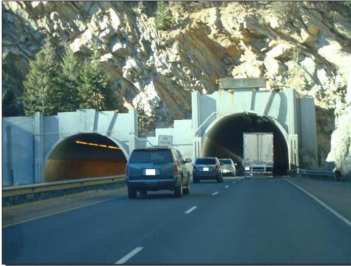
WESTBOUND APPROACHING THE TWIN TUNNELS
