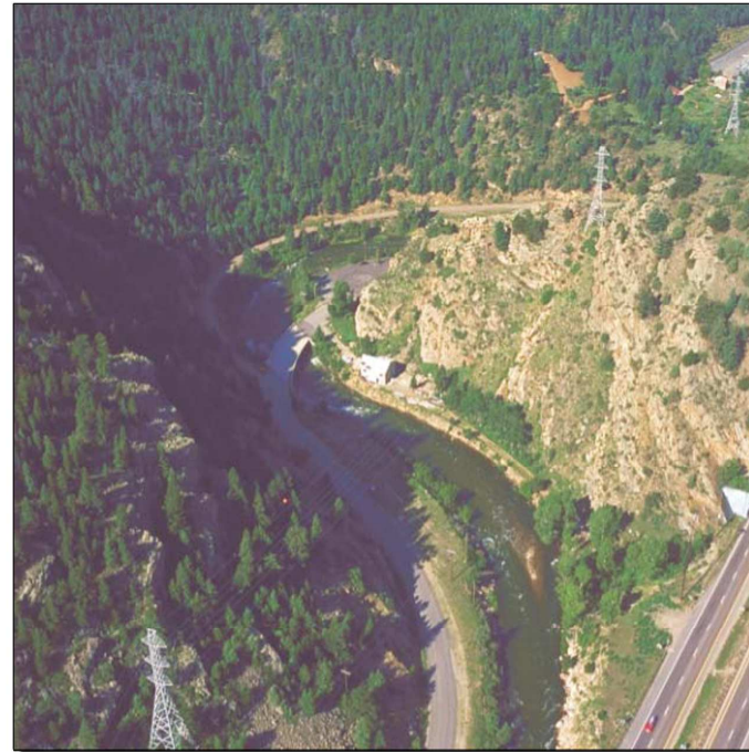
VIEW OF SOUTHSIDE OF TWIN TUNNELS - FROM LEFT TO RIGHT: IDAHO SPRINGS ROAD E, CLEAR CREEK, AND I-10
