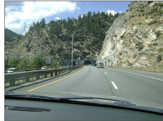
WESTBOUND APPROACHING THE TWIN TUNNELS
