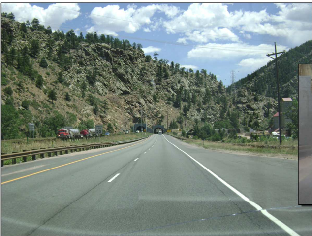
EASTBOUND APPROACH TO TWIN TUNNELS FROM IDAHO SPRINGS
