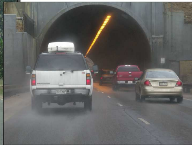
EASTBOUND ENTERING THE TWIN TUNNELS
