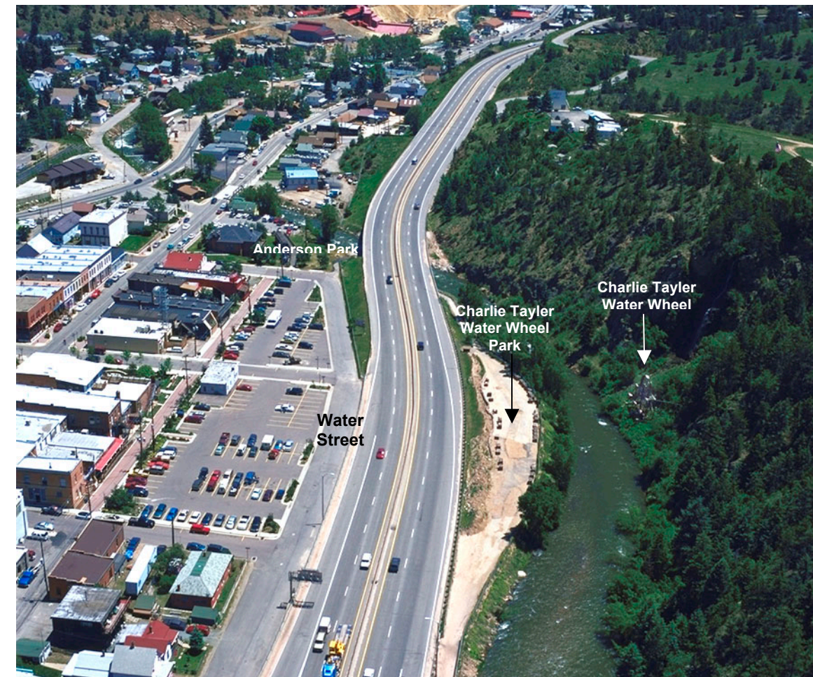
Figure 3.16-13. Oblique View of Charlie Tayler Water Wheel Park
