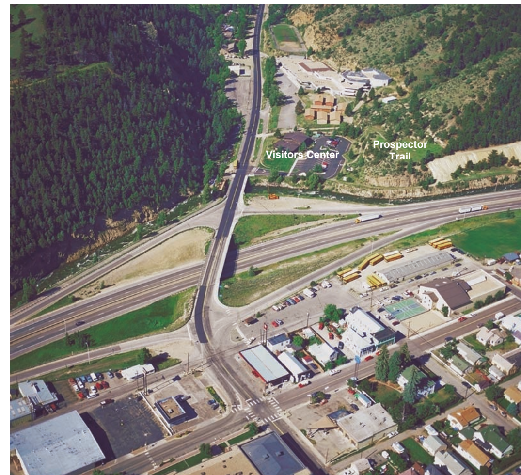
Figure 3.16-10. Oblique View of USFS Visitors Center (Clear Creek District) and Prospector Trail
