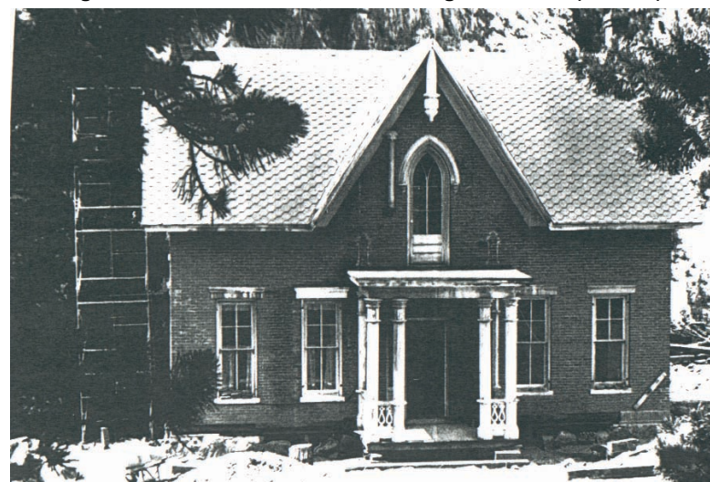
Figure 3.16-3. Toll House, Mine Manager's House (5CC.13)
