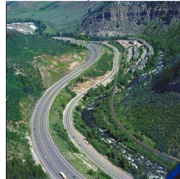
View West at Dowd Canyon milepost 171
