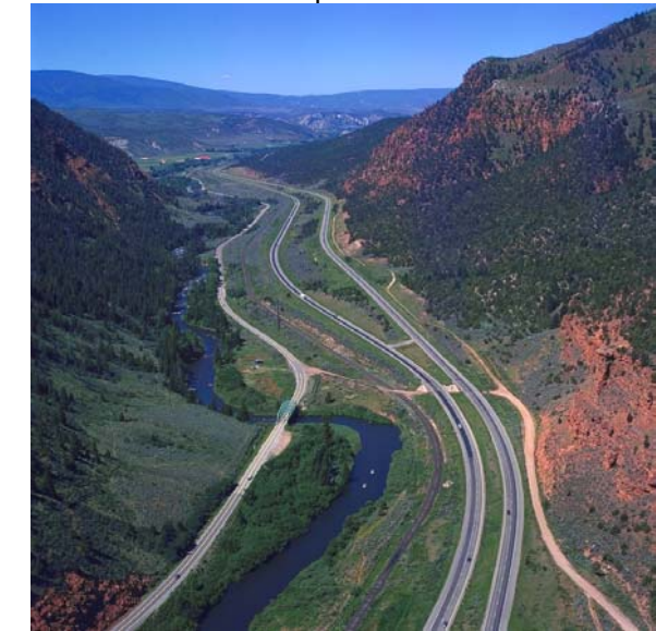
View West over Red Canyon milepost 152
