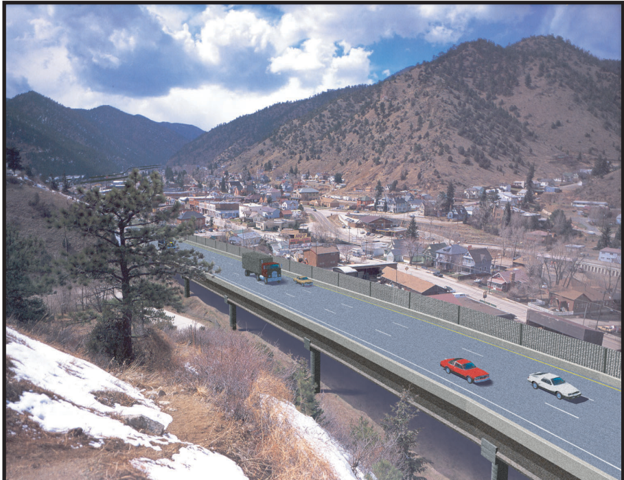
6-LANE HIGHWAY ALTERNATIVE WITH SOUND WALL MITIGATION SIMULATION (Please note that sound walls are one possible future option)
