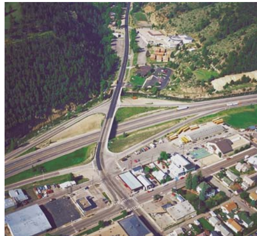
Oblique View of USFS Visitors Center (Clear Creek District) and Prospector Trail
