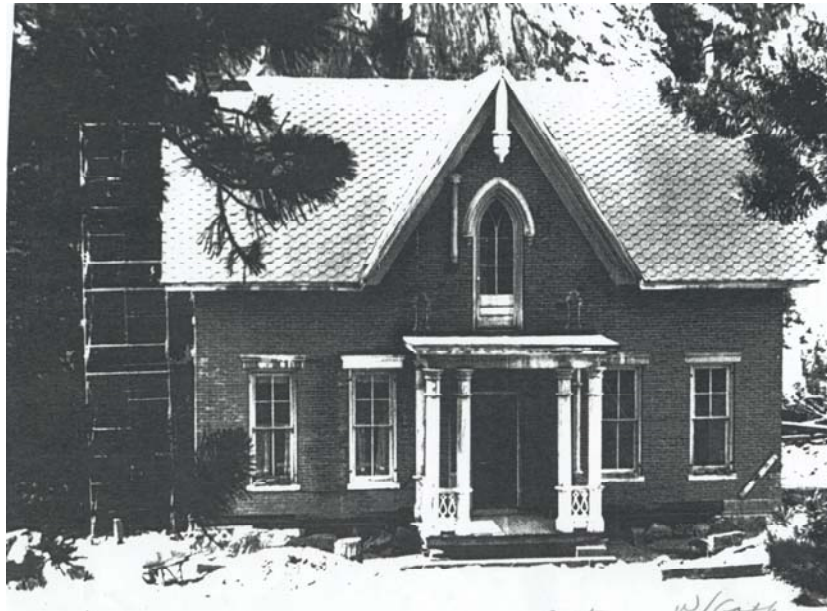
Toll House, Mine Manager's House (5CC.13)
