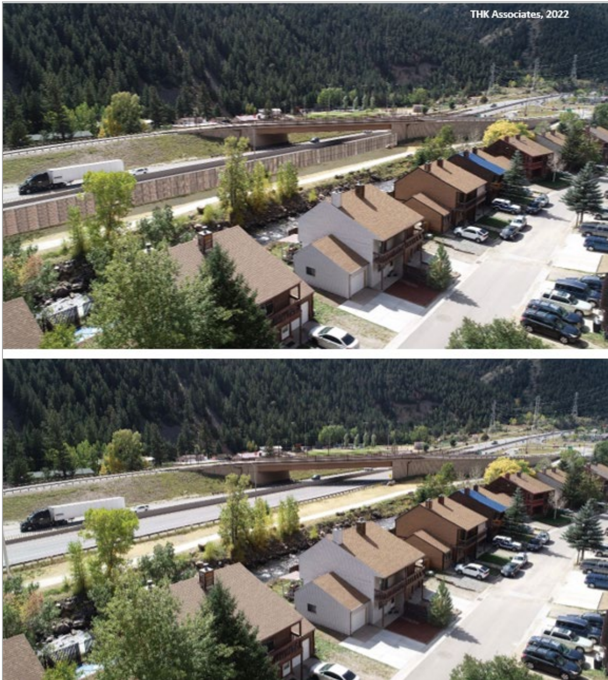
Proposed Noise Wall in eastern Idaho Springs (top) will benefit 28 residences that are impacted by traffic noise higher than FHWA noise abatement criteria (bottom picture is existing condition).
