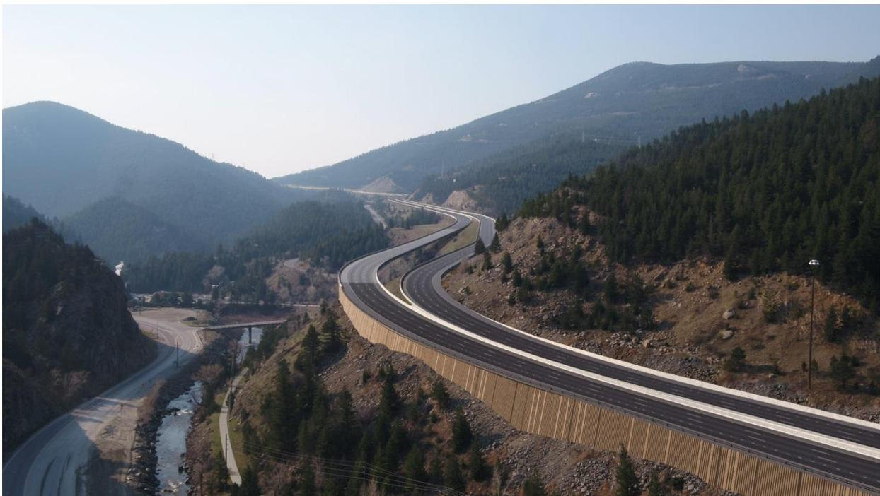
In this photograph, I-70 WB is widened from 2 lanes to 3 lanes to accommodate more WB travelers. I-70 will be reconfigured to simplify curves, improve site distance and safety.
