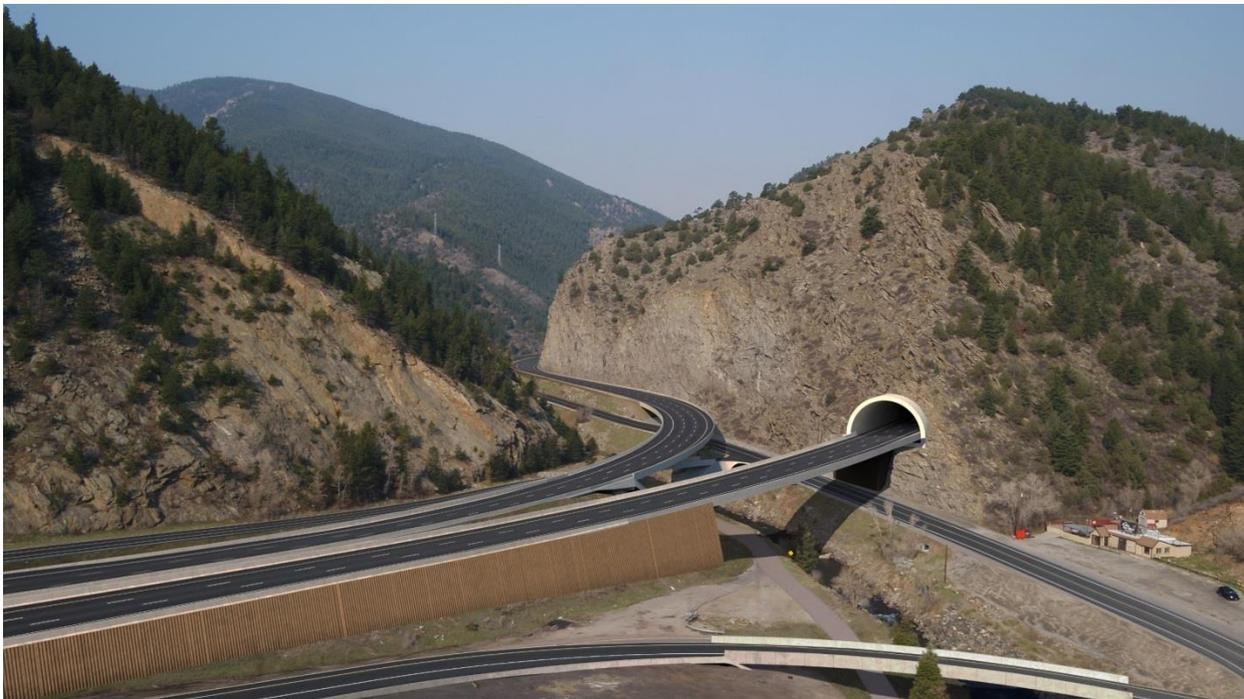
At I-70 and US 6, the project will maintain the existing WB I-70 exit-ramp and add an EB I-70 on-ramp. US 6 will be extended to the west providing additional access to and from I-70 at the Hidden Valley interchange with Central City Parkway and will connect with CR 314. WB will be placed in tunnel. Greenway trail will be improved from US 6 to VMT.
