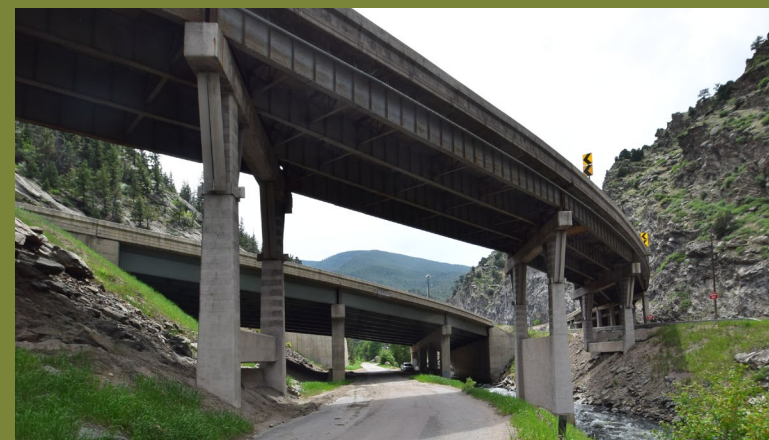
The westbound I-70 bridge at the bottom of Floyd Hill is structurally and functionally deficient and needs to be replaced whether or not the Project is approved.
