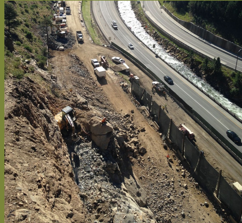
Source: Kraemer North America construction of westbound Twin Tunnels, 2014.
