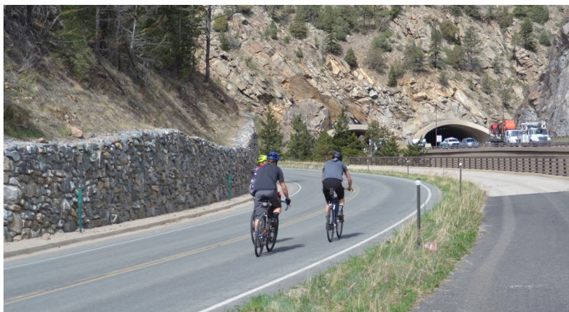
Exhibit 4-2. Existing Retaining Walls along CR 314 that will be Replaced after New Rock Cuts to the South
