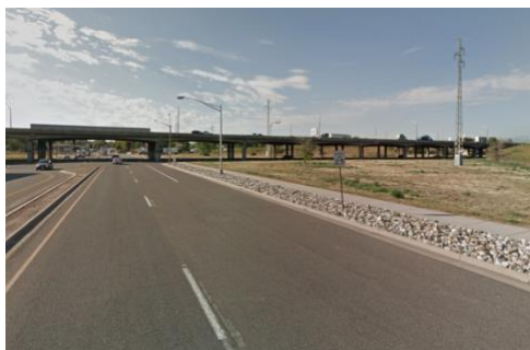
Steele Street before construction in 2014.
