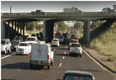
Peoria Street before construction in 2017.
