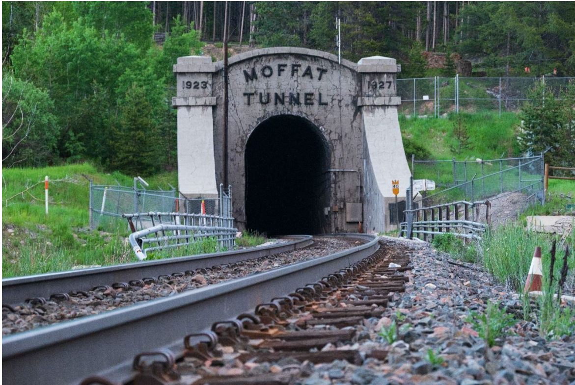
Figure 21: West Portal of the Moffat Tunnel
