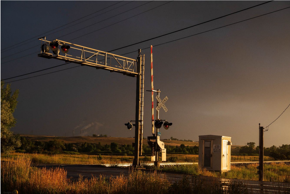
Figure 23: Grade Crossing in Craig, CO
