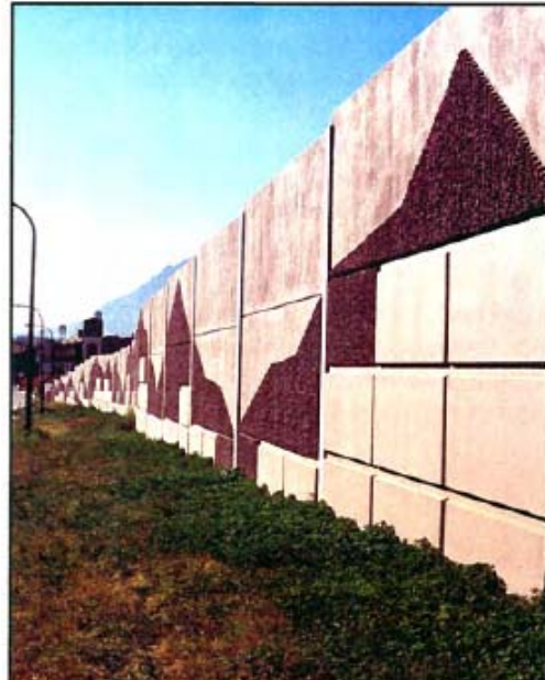
Exhibit 4-9. Example of CDOT Noise Wall in Colorado Springs
