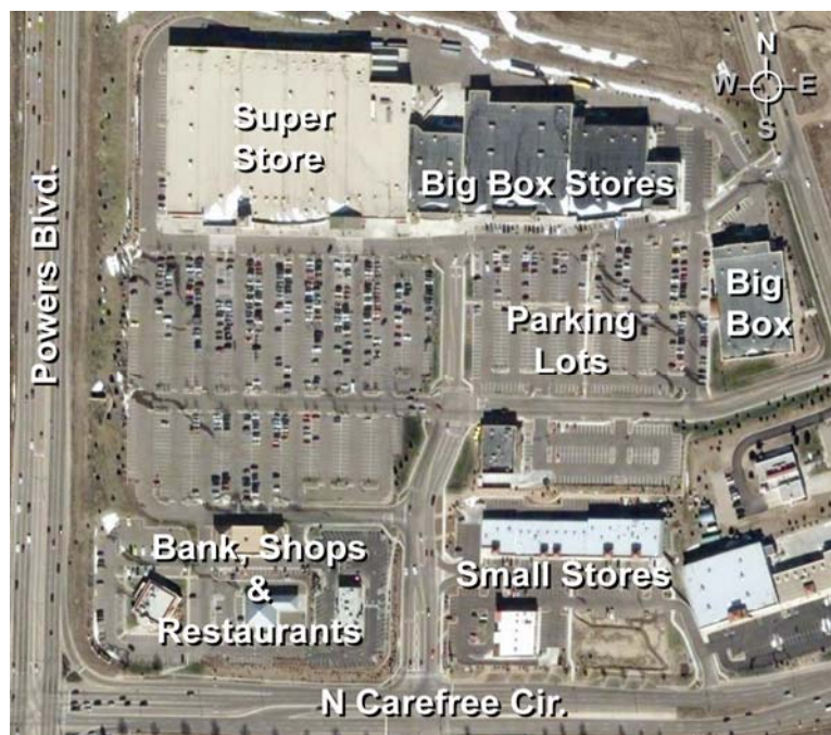
Exhibit 2-7. Intense Retail Development Adjacent to a Powers Boulevard Intersection
