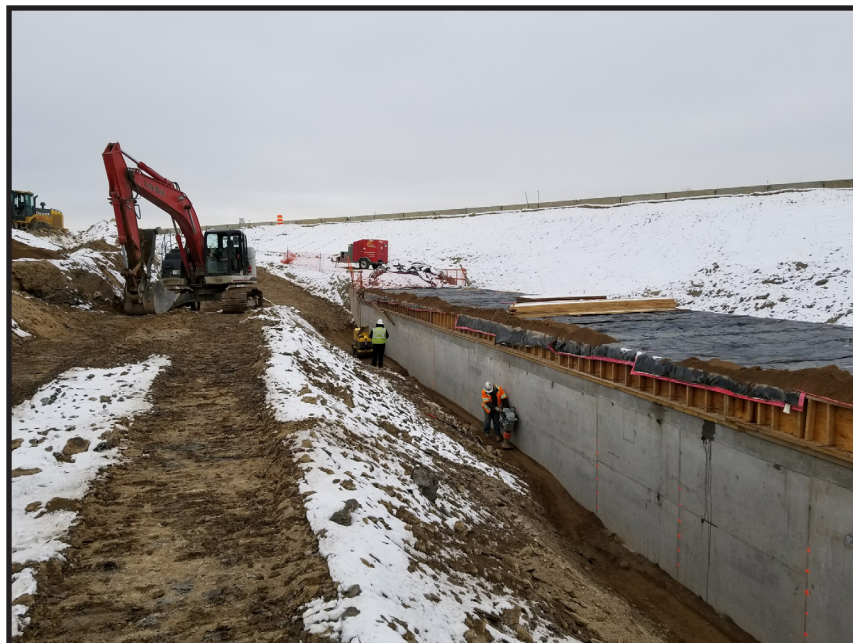
Work crew is backfilling the concrete box culvert.
