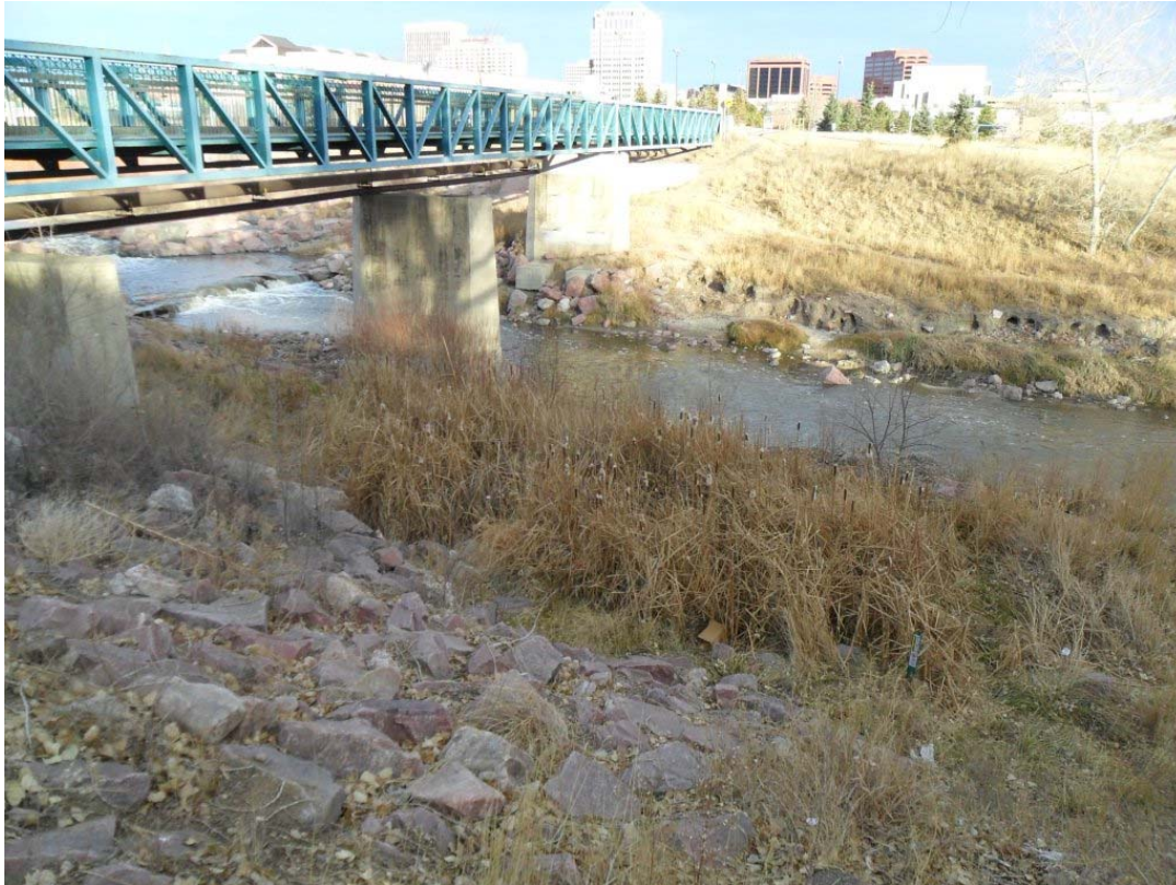
Photo 6: View of Wetland 2 on terrace adjacent to Monument Creek and under a pedestrian bridge. Wetland is dominated by cattails.
