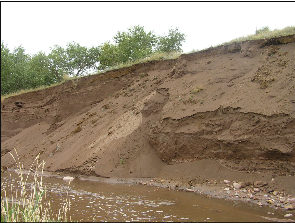
Photo 3. Bank erosion along Fountain Creek, Colorado Springs, Colorado.
