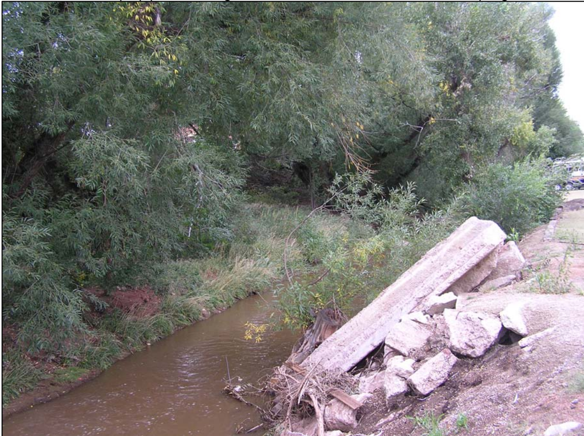
Photo 2. Concrete riprap present along the banks of Fountain Creek, Colorado Springs, Colorado.
