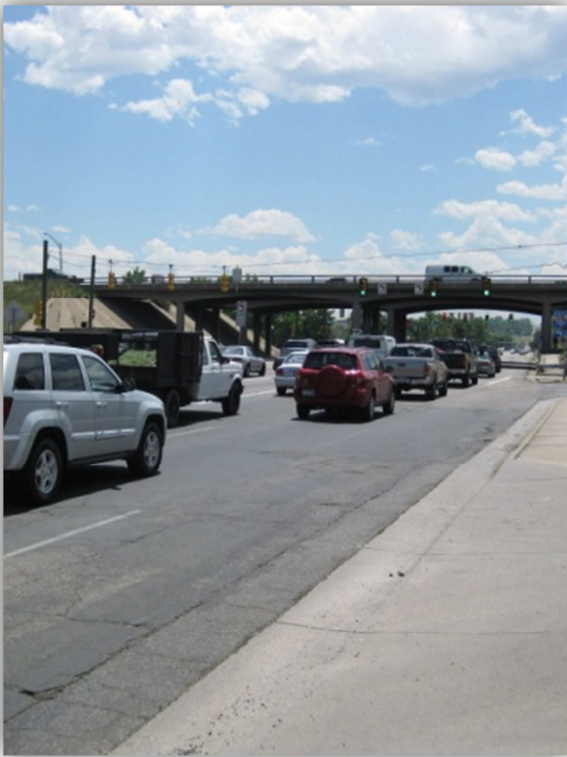
Kipling Street at eastbound I-70 ramps intersection
