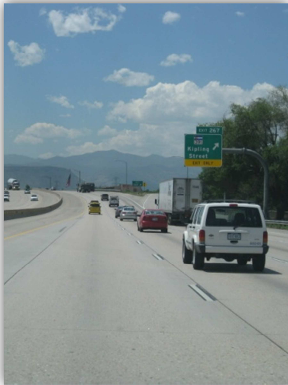
Westbound I-70 approaching Kipling interchange
