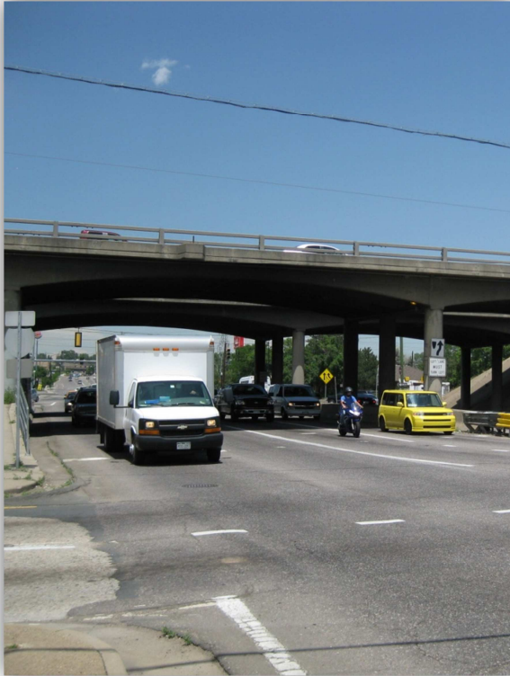
Looking north along Kipling Street towards I-70
