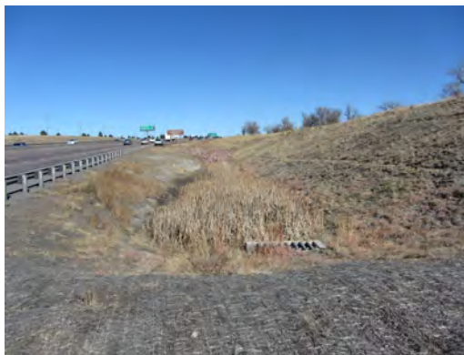
Photo #23: New WQ Pond (East I-25)
