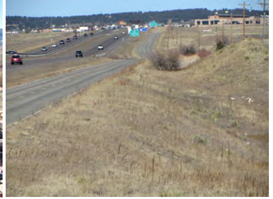
Photo #2: B -Teachout Creek (East I-25)
