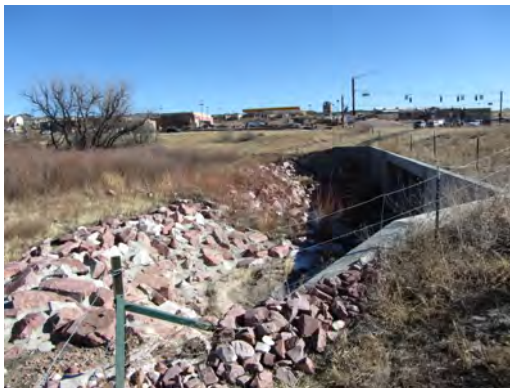
Photo #7: AZ -Jackson Creek (North Baptist Rd.)
