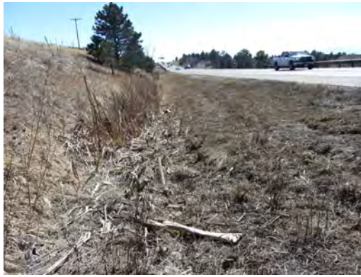
Photo #17: W Roadside Swale (East I-25)
