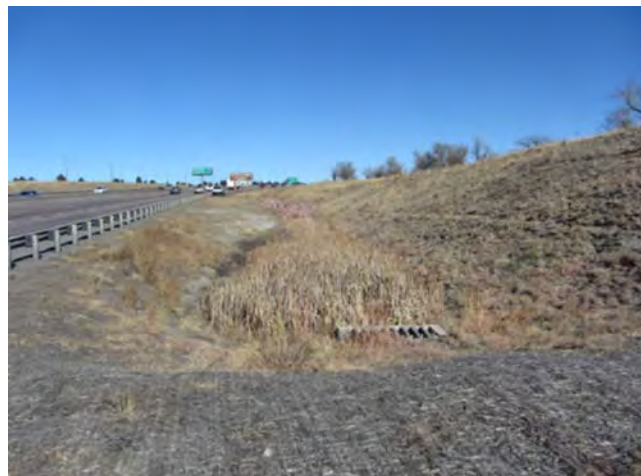
FIGURE 2. New Wetland on the Eastern Side of I-25, South of Exit 150
