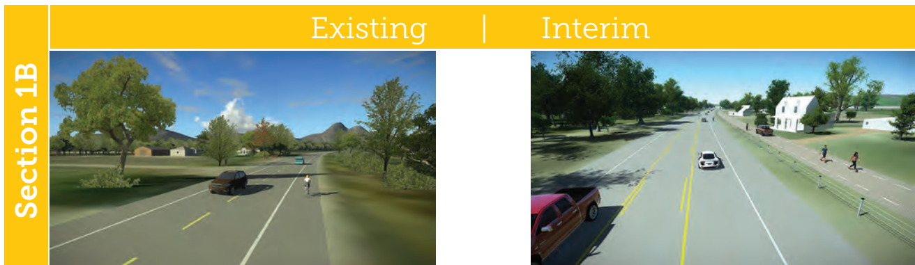
No median separation or left turn lanes
