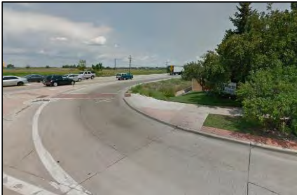
Lack of sidewalks on SH 66: Hover St/SH 66 and Pace St/SH 66 - Sidewalk connections provided south of SH 66, but not extended along SH 66
