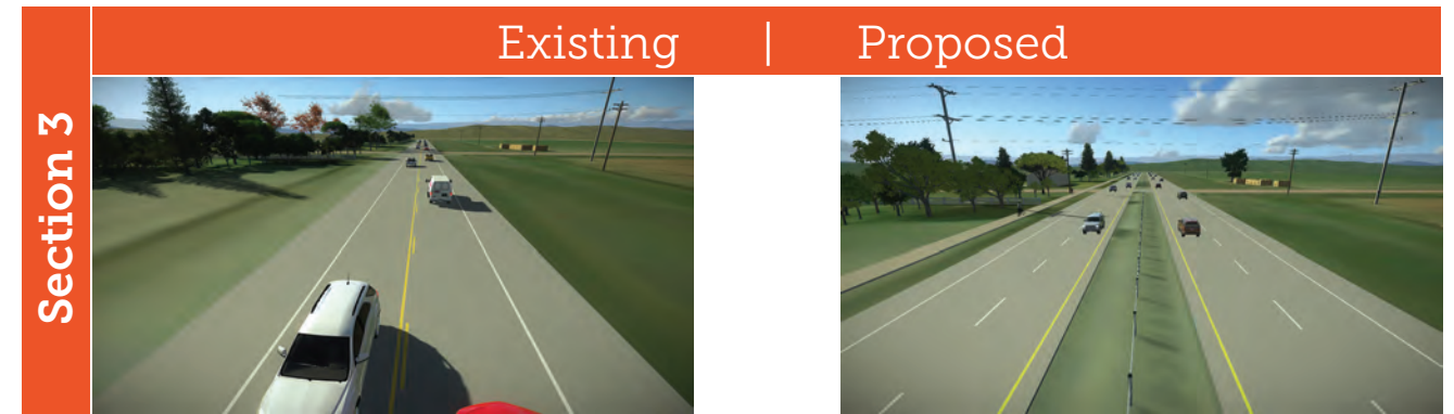
No median separation or left turn lanes
