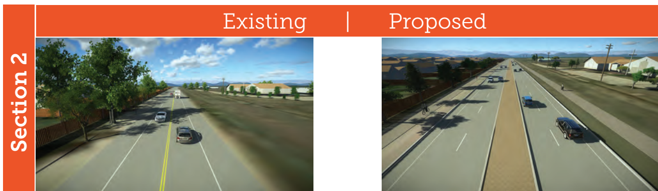
No median separation or left turn lanes
