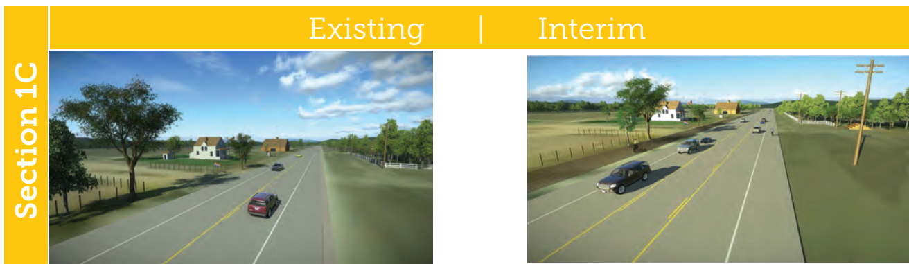
No median separation or left turn lanes
