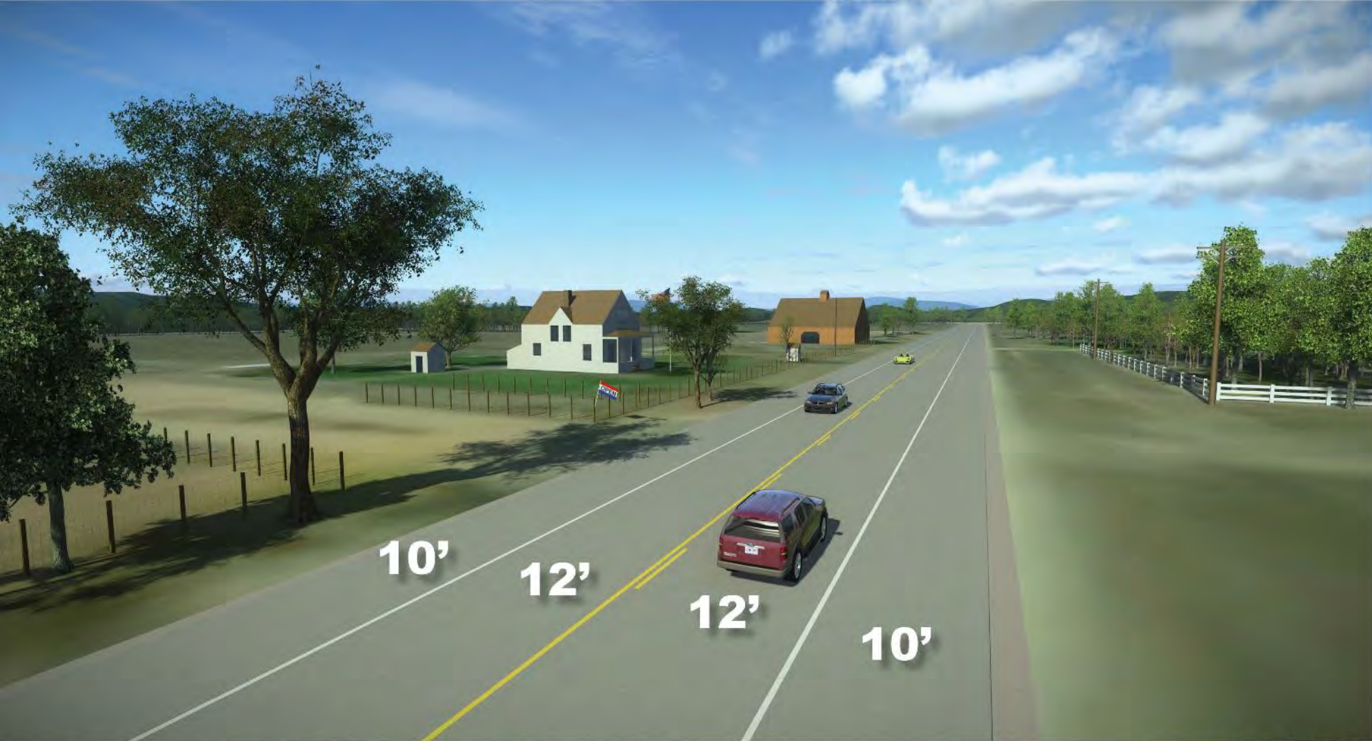
Section 1C - existing roadway conditions
