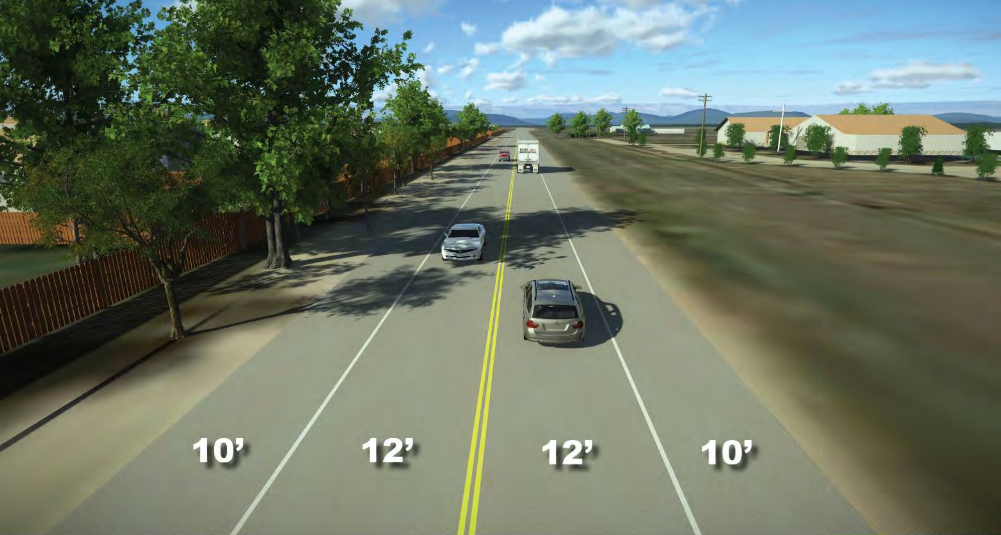
Section 2 - existing roadway conditions
