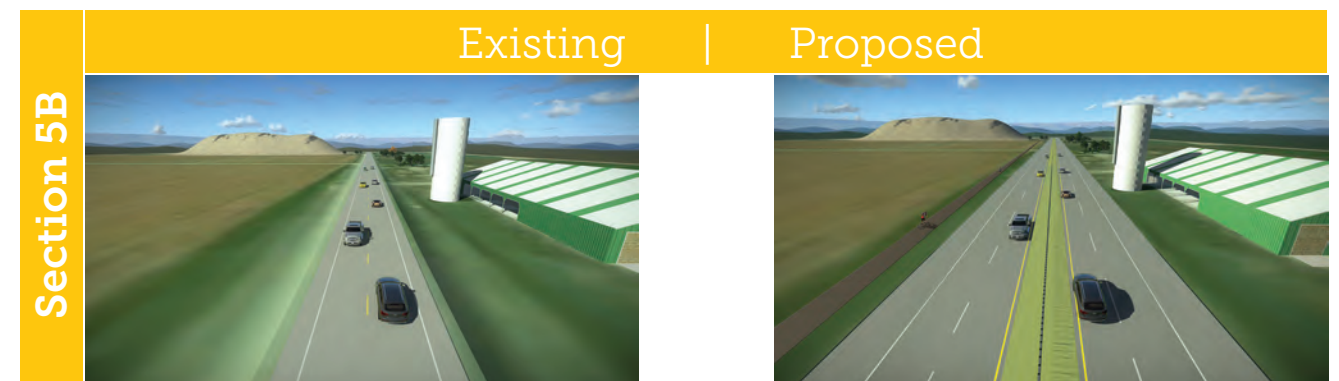
No median separation or left turn lanes
