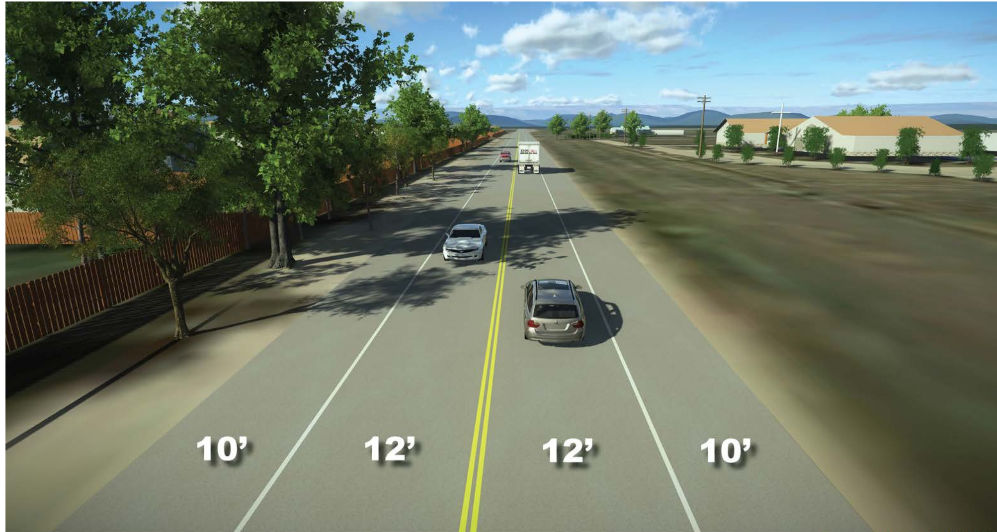
Section 2 - existing roadway conditions
