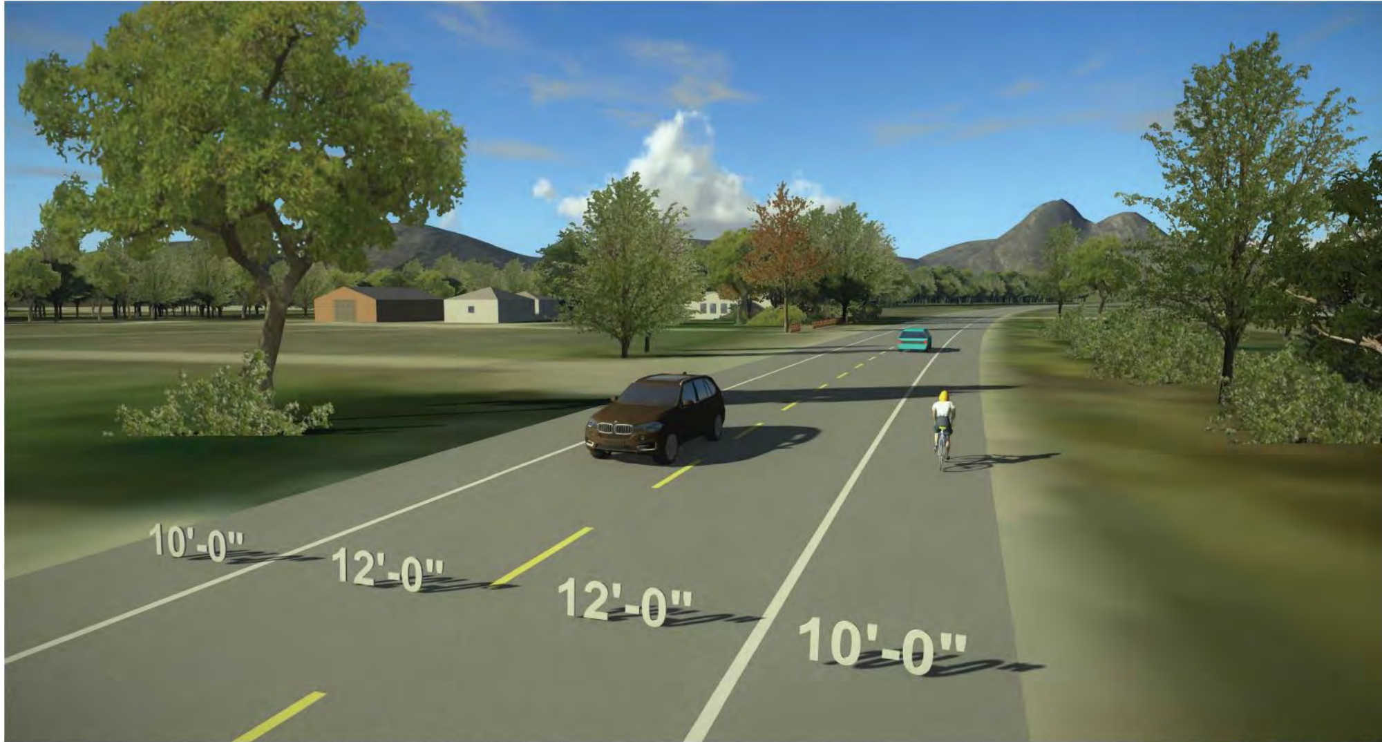
Section 1B - existing roadway conditions
