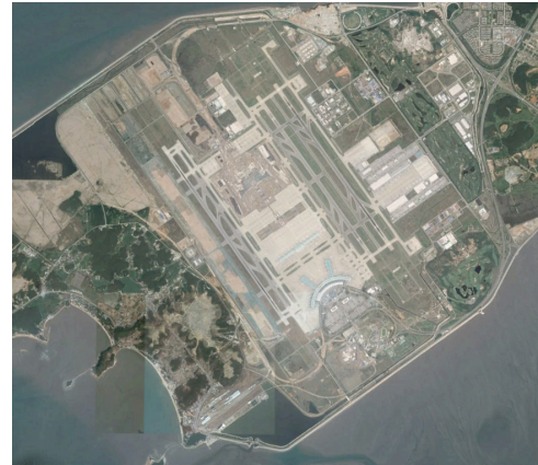
Incheon International Airport/Songdo International Business District, Seoul, Korea
