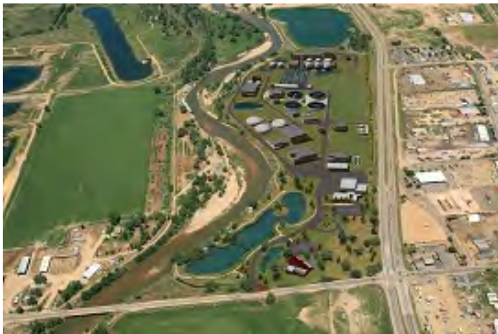
MWRD Northern Treatment Plant
