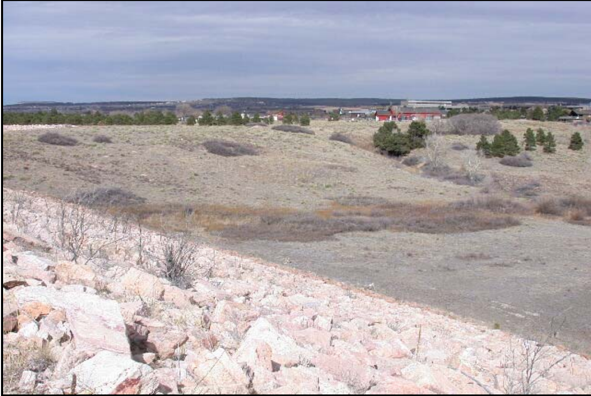
Photo 15. Looking north from the top of the Kettle Creek dam on the east side of I-25. Note the diagonal drainage at the top right of the photo with heavy shrub cover. If Preble's can move through this area and over the dam, a new culvert could be installed under I-25 that would allow movement under the highway. 11/07/02.
