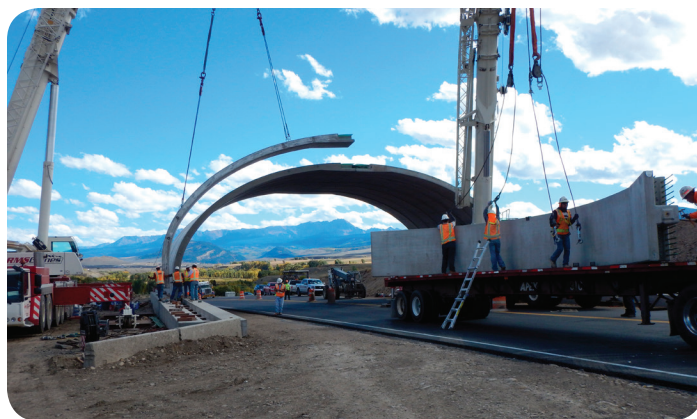
Crews work to complete precast concrete structures
