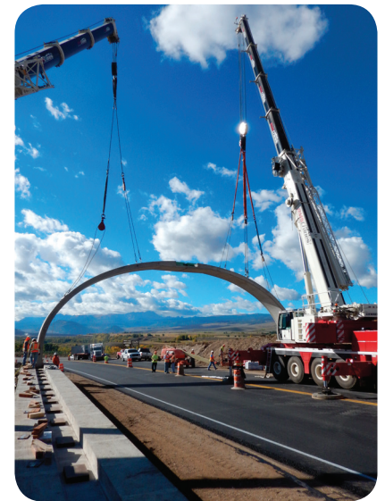
Construction cranes used to install overpass arch
