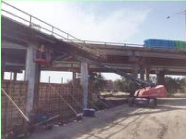
*Falsework used on the new two-span I-25 bridge over Union Pacific Railroad tracks*
