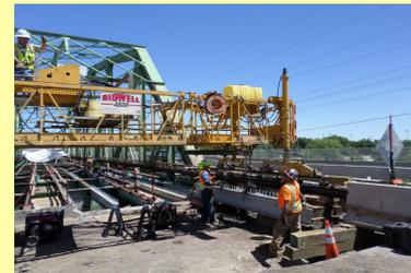
*Engineered Bidwell working as a gantry crane*
