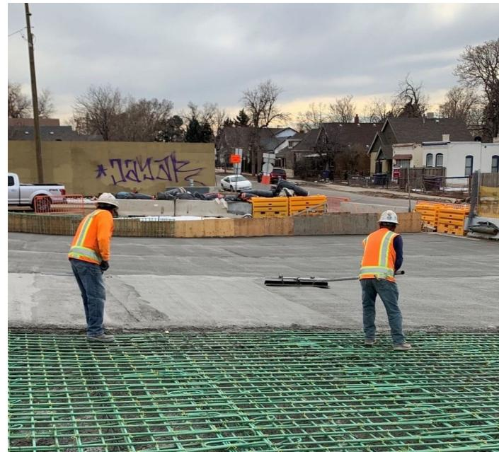
In February, the Central 70 Project completed the last concrete pour on the cover park deck. There were more than 3,000 cubic yards of concrete poured! Along with the concrete pour, crews have installed the last drilled shaft, which are deep foundation solutions to support heavy loads, for the cover park structure. This critical work allows the crews to begin construction of the Swansea Elementary School playground, along with the
