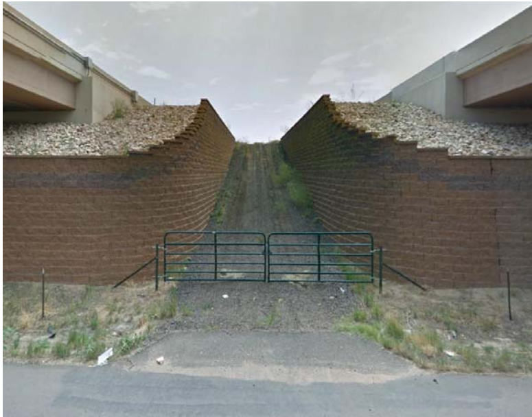
Figure 2.9 Example of I-25 median access between bridges at WCR 20
