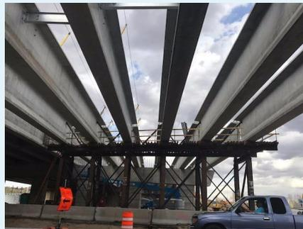
I-25 bridge girders are precast concrete beams and vary from 72 to 155 feet in length and are an integral part of the bridge deck support structure that carries the traffic. A 500-ton and a 300-ton capacity crane were used
