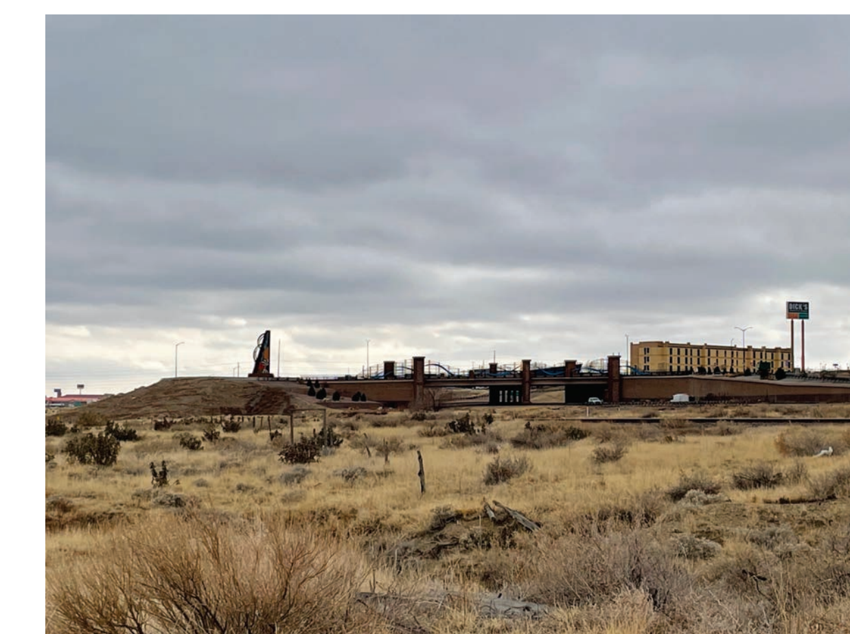
Looking southwest towards the future I-25 east frontage road bridge location and tie-in at Dillon Road
