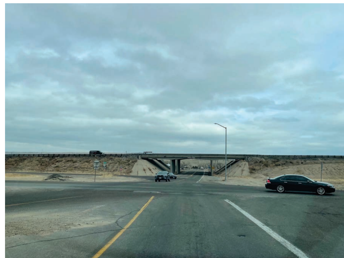
Existing Drew Dix Parkway and I-25 west frontage road intersection where a roundabout will be constructed
