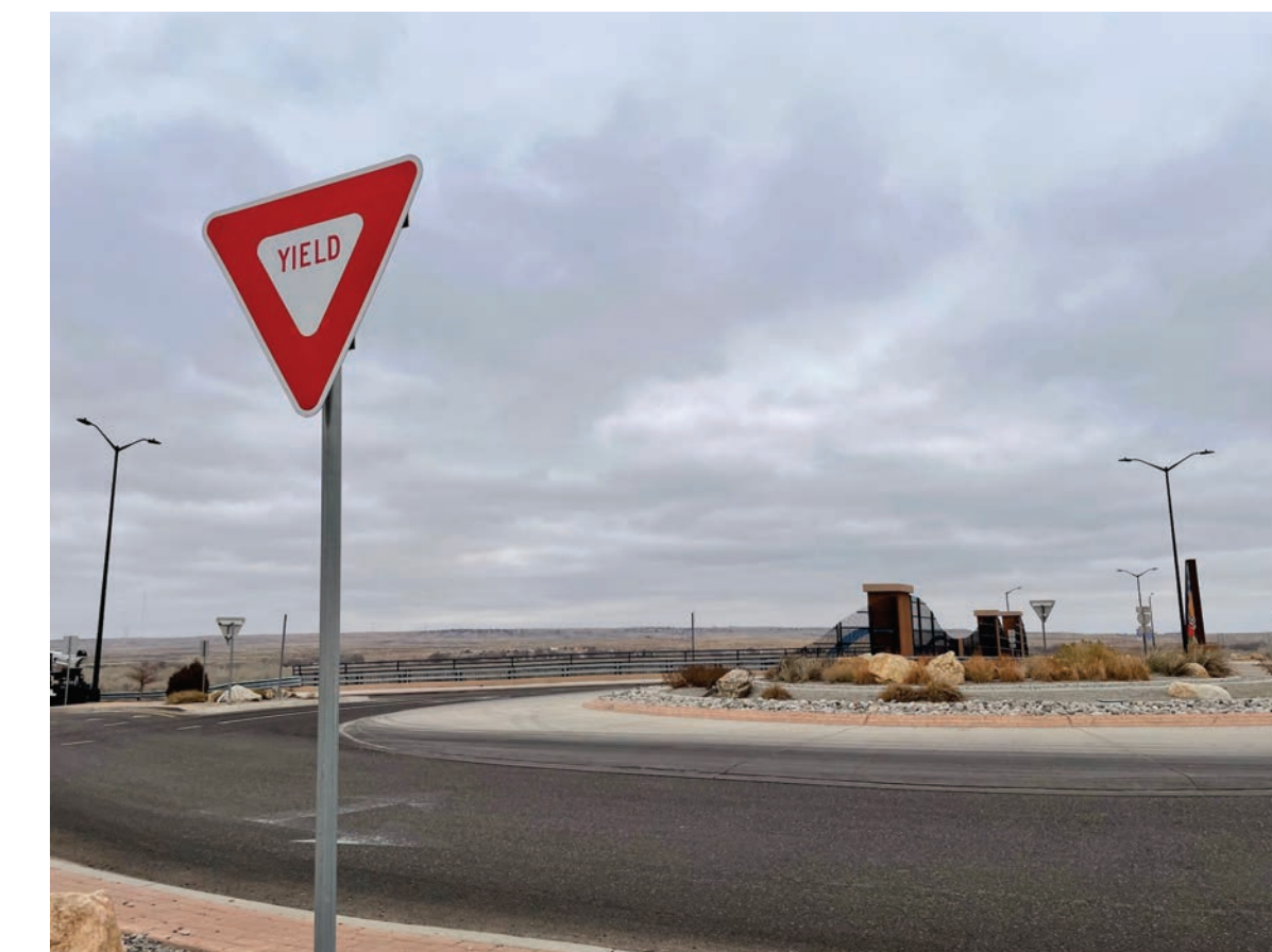
Existing roundabout at Dillon Drive and the I-25 west frontage road
