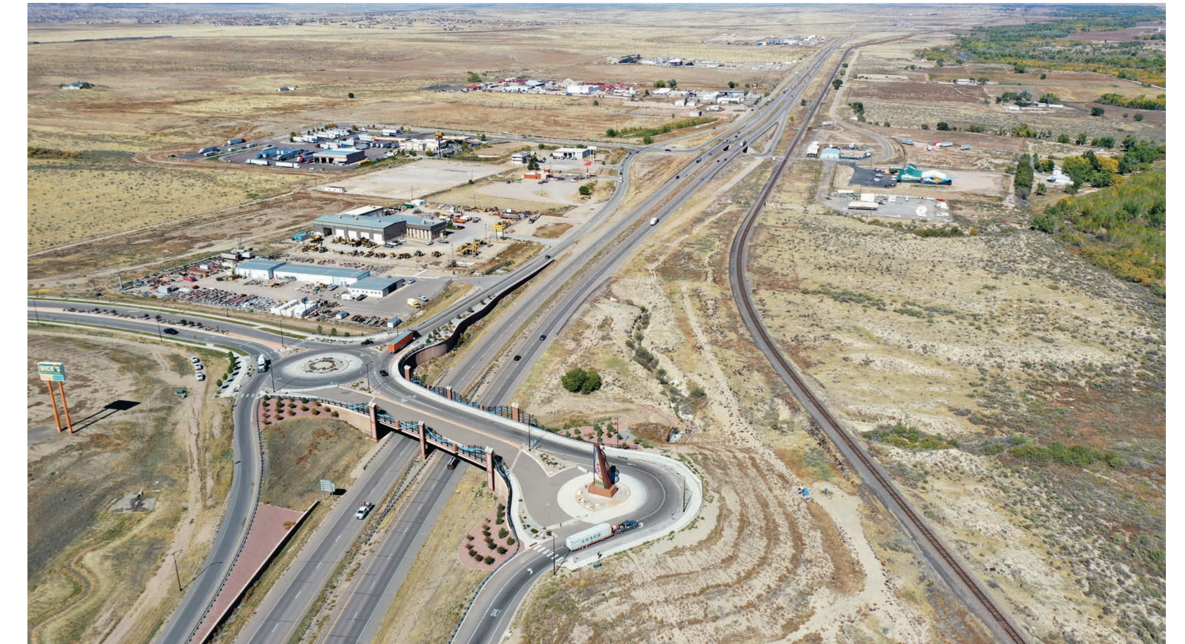
Looking north along future I-25 east frontage road alignment at Dillon Drive
