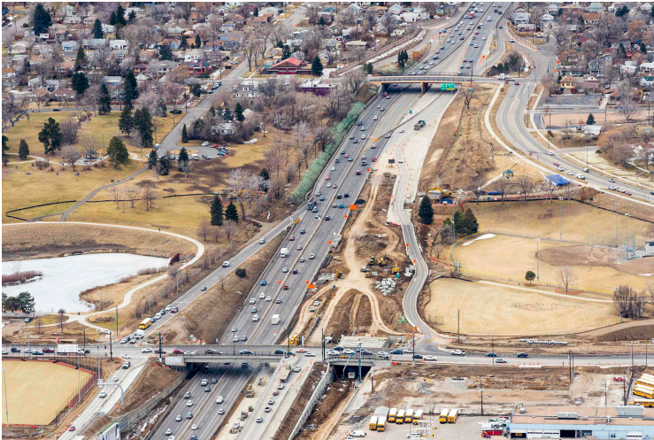
Looking west at the Federal and Knox bridges over US 6
