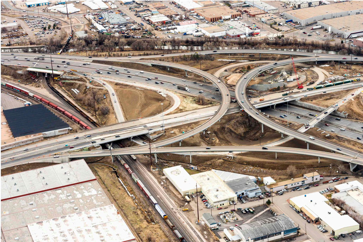
US 6/I-25 Interchange
